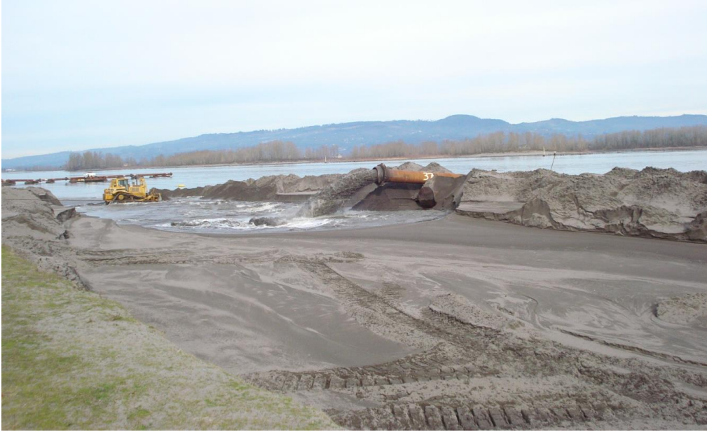
Figure 8 Active shoreline placement at Sand Island (looking downstream)
