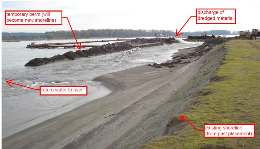
Figure 6 Active shoreline placement at Sand Island (looking upstream)
