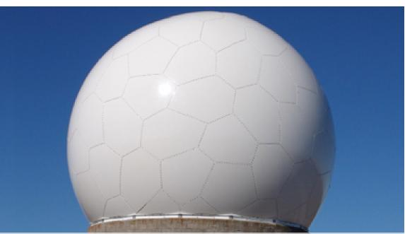
Research and development conducted by Infinite Technologies, Inc. under the Air Force Small Business Innovation Research and Small Business Technology Transfer Program managed resulted in an advanced composite radome technology. (Courtesy photo)
