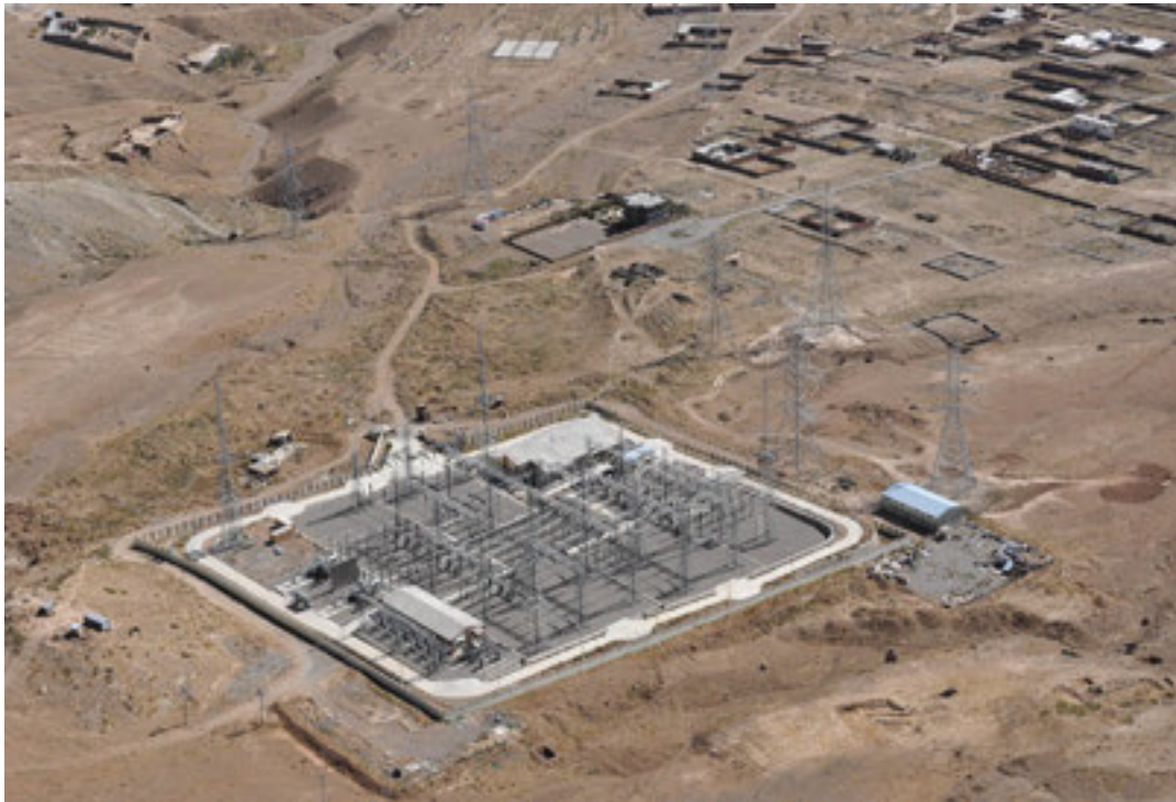
U.S. Army Corps of Engineers along with a team of program managers and engineers, conducts aerial inspections of Charikar Substation, power lines and other project sites. (DoD photo)
