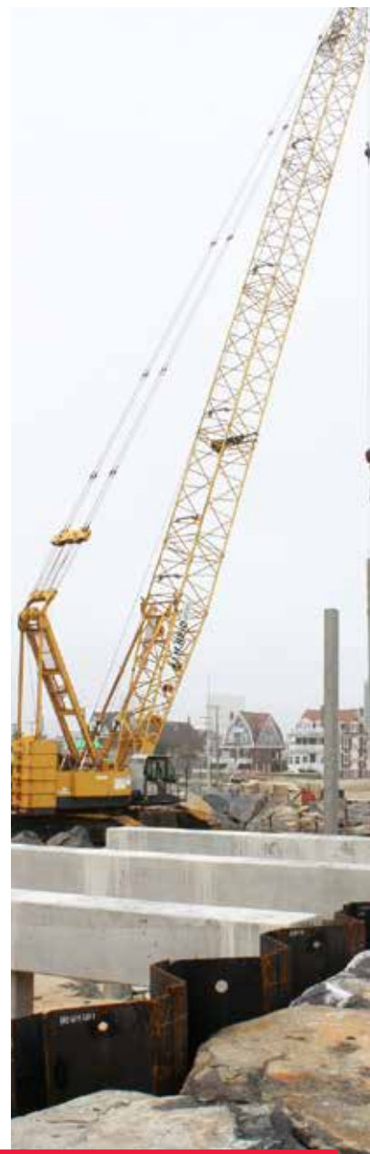
PHILADELPHIA DISTRICT AND ITS CONTRACTOR BUILDING TWO SECTIONS OF A SEAWALL (U.S. ARMY CORPS OF ENGINEERS PHOTO BY TIM BOYLE).
