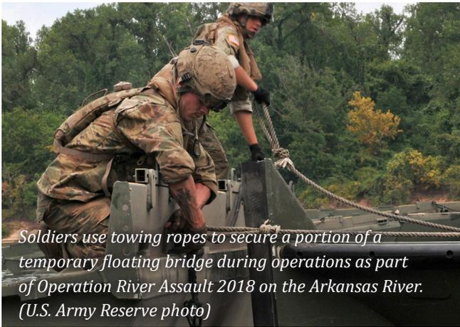
*Soldiers use towing ropes to secure a portion of a temporary floating bridge during operations as part of Operation River Assault 2018 on the Arkansas River. (U.S. Army Reserve photo)*
