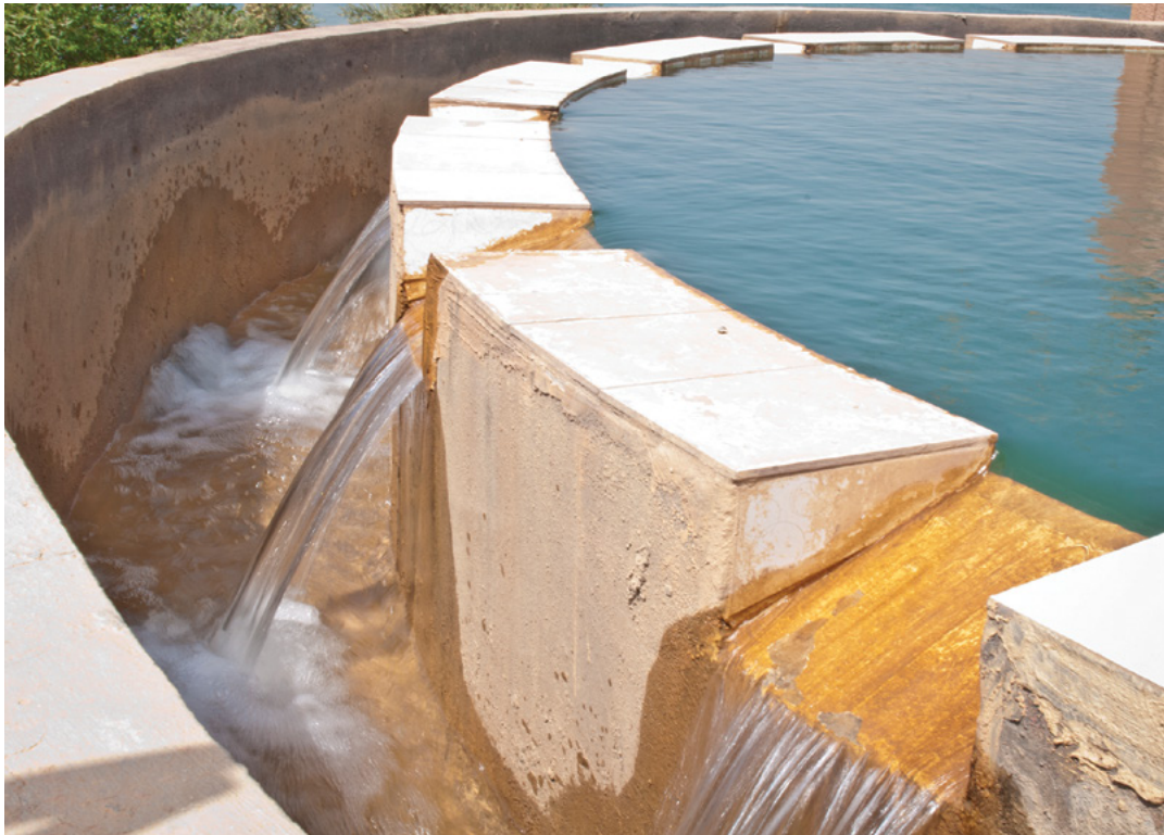
Water flows through a collection tank at the Al-Awghi Water Pumping Station in Shahil, Syria, one of the few currently operational in the region. (U.S. Army photo)
