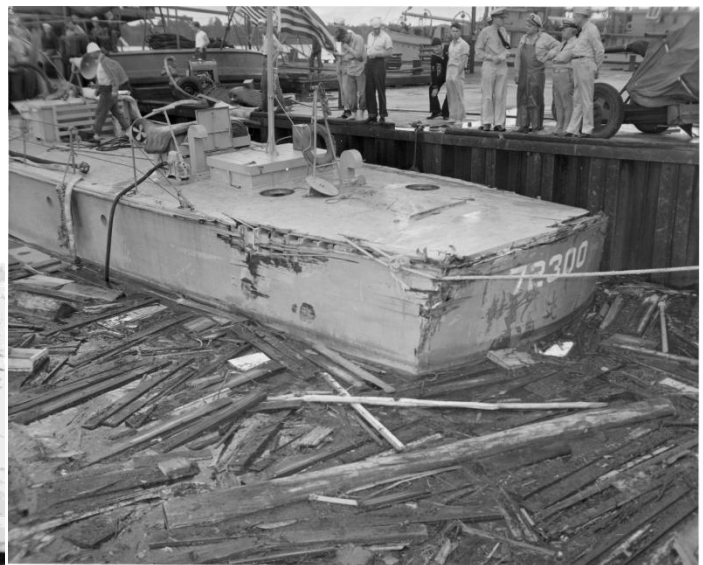
CG-72300 damage in storm at Little Creek, VA 14Sep44
