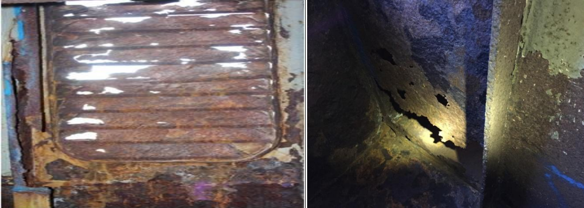
Figure 28. Photographs taken by Coast Guard Traveling Inspectors during an October 2016 visit to EL YUNQUE in Tacoma, WA showing examples of corrosion within the vessel’s exhaust ventilation trunks. (U.S. Coast Guard photographs)
