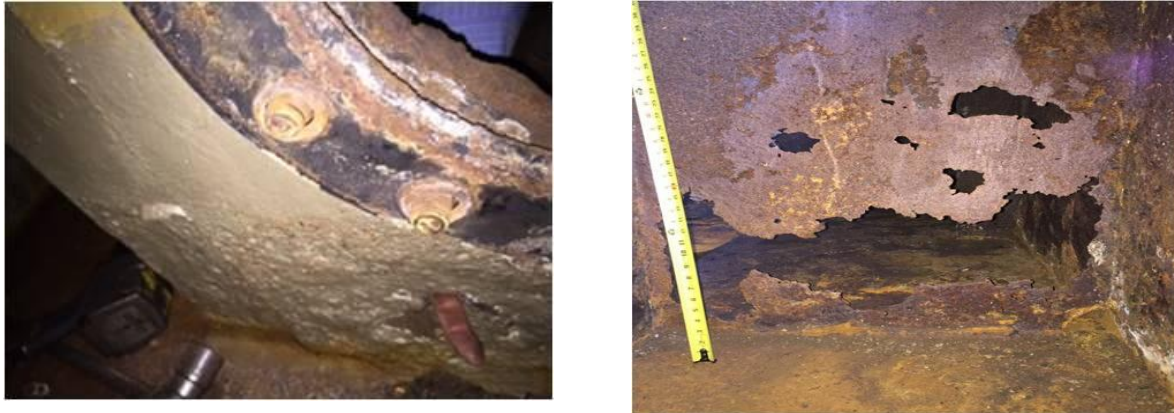
Figure 27. Examples of wastage found within an EL YUNQUE ventilation trunk that were found by Coast Guard Traveling Marine Inspectors during a February 1, 2016, DOC audit of TOTE.
