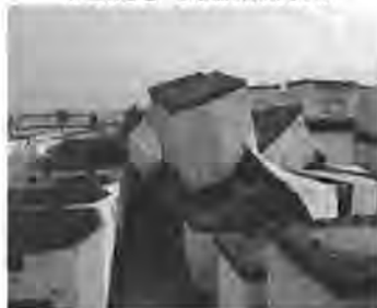
Figure 5. Collapsed JLIST Containers
