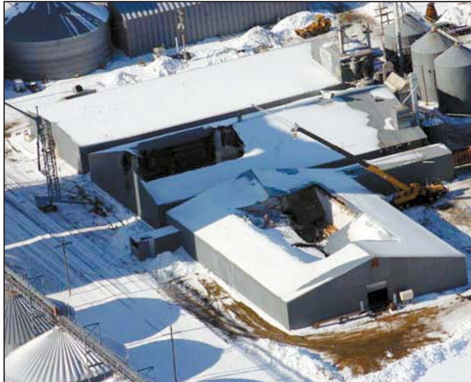
Collapsed roofs on these farm buildings give witness to the destructive power of the winter storm that dumped snow on much of Western and Central Kansas in late December 2006. (Photo provided by Kansas Highway Patrol)
