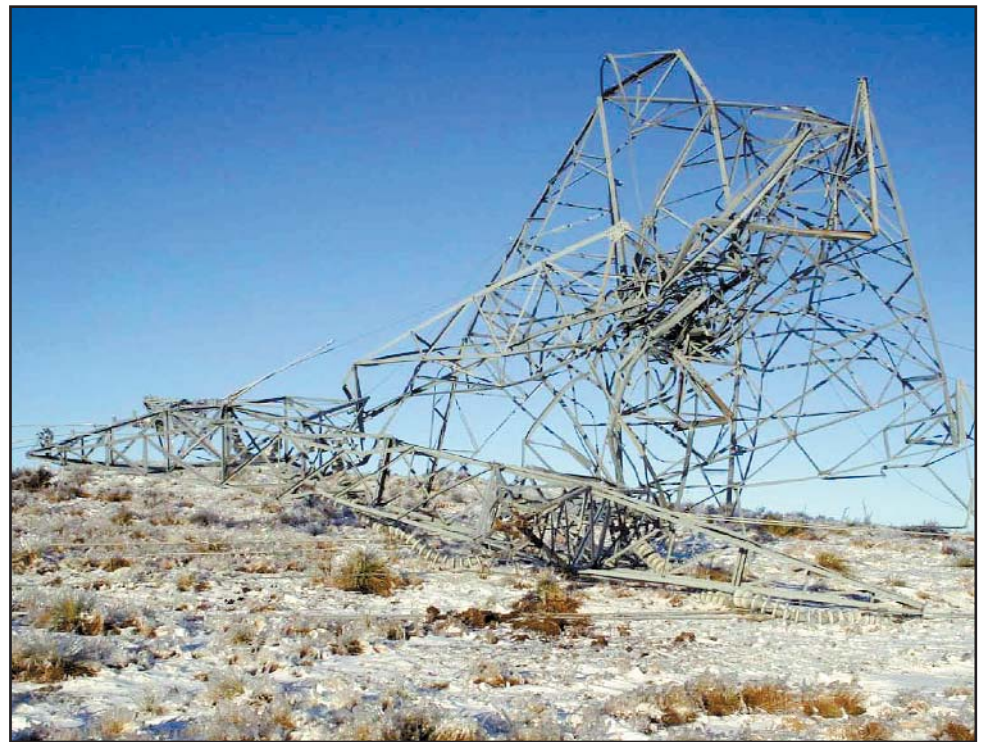
Steel electrical transmission towers lie in twisted ruins in Grant County, the victims of a powerful winter storm that swept into the state in late December 2006. The storm covered the western half of the state with ice and snow, knocked out power to more than 60,000 customers and left cattle stranded in the fields. (Photo by xxxx)
