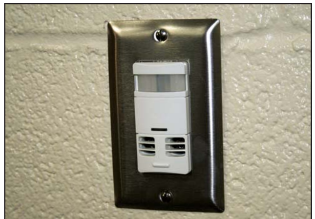
Occupational sensor switches have been installed in state armories to help reduce electrical costs.
