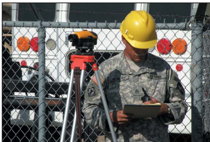
Staff Sgt. Kevin Murphy, 242nd Engineer Company (Horizontal), checks his numbers while surveying the Salina Unit Training Equipment Site expansion work site to see if more cut or fill would be needed.
