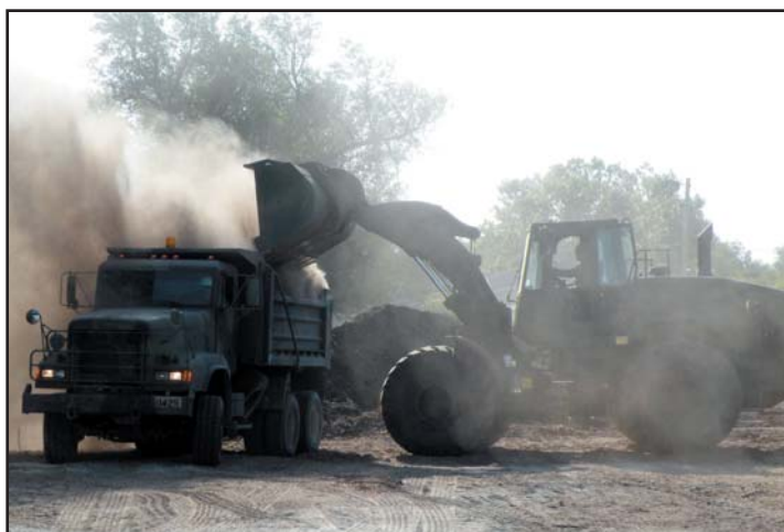
A front loader dumps dirt into a 20-ton dump truck during the Unit Training Equipment Site expansion project in Salina.
