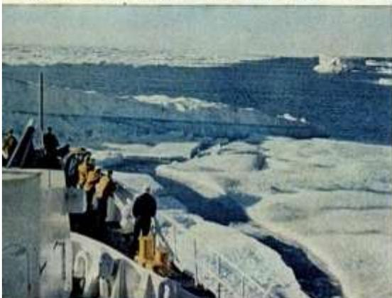
**ICE-PACKED PORTRAIT** of *Northwind* is taken by crew member. Icebreakers are broad and stubby, have reinforced hulls for riding up on ice and cracking it.
