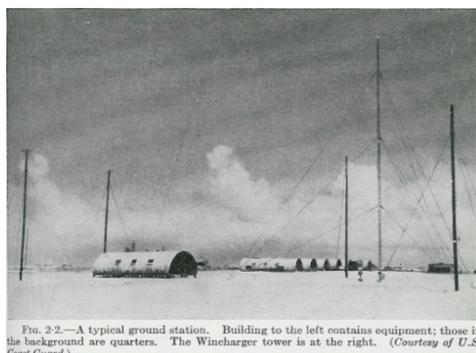
FIG. 2.2.—A typical ground station. Building to the left contains equipment; those in the background are quarters. The Winch tower is at the right. (Courtesy of U.S. Coast Guard.)
