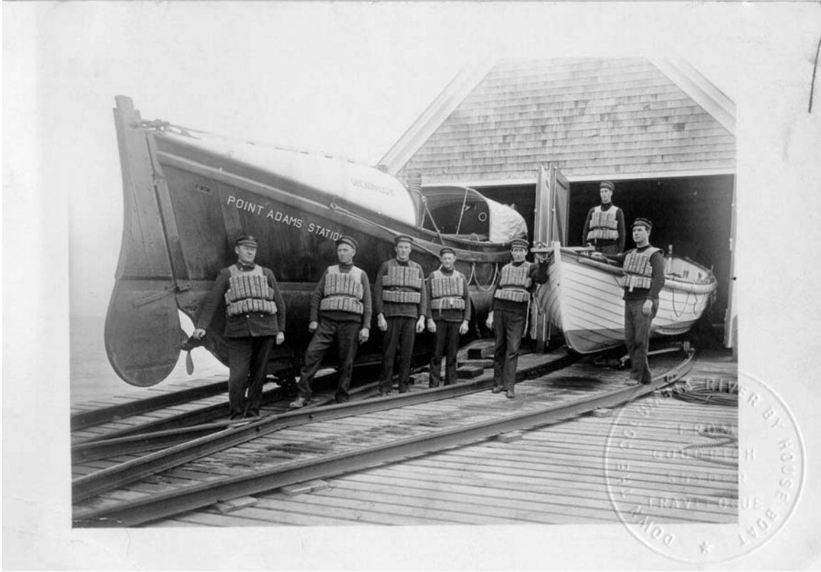
"Point Adams Sta. Boat House Launching Station No. 311." Postcard photo stamped: "SUPT. OF CONSTRUCTION & REPAIR OCT 23 1916"; stamped in bottom right corner: "Down the Columbia River by House Boat: From Goodrich Synder Travelogue." No other information noted.
