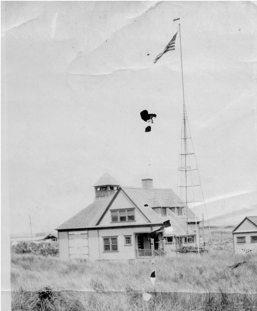
"Coast Guard Station No. 90, Long Beach, N.Y.; built in 1889 (R.J.L.); destroyed by fire, Dec. 9th, 1917, (R.J.L.)."; photo dated 24 September 1917; no photo number; photographer unknown.
