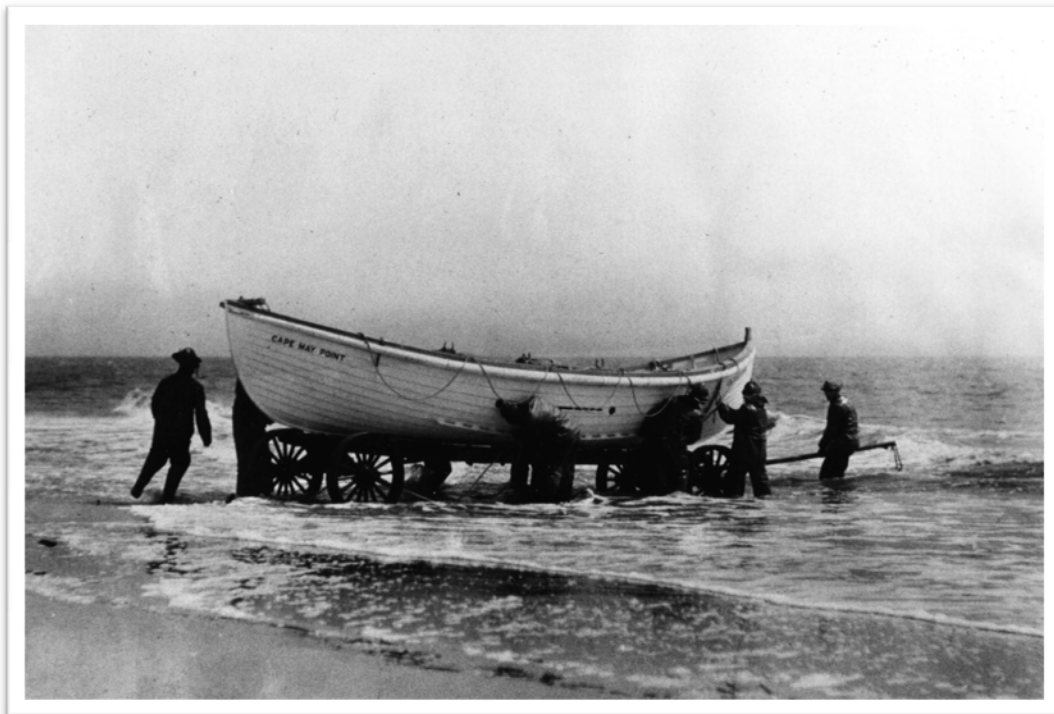
No caption/date/photo number; photographer unknown. The pictured surfboat is the 25-foot Type S pulling surfboat No. 4435/CG25419. It was built in 1934. Photo courtesy of Van Field; information regarding the surfboat was provided by Tim Dring.
