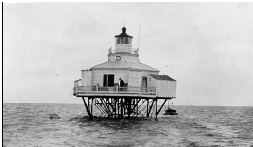
Figure 3-14. Post-1911 photograph of the Halfmoon Reef Lighthouse. Note the steep roof and the absence of the second story deck, the results of the extensive alterations made in 1911. Two water cisterns and two storage sheds or outhouses are built on the deck surrounding the main floor (United States Coast Guard 2009).
