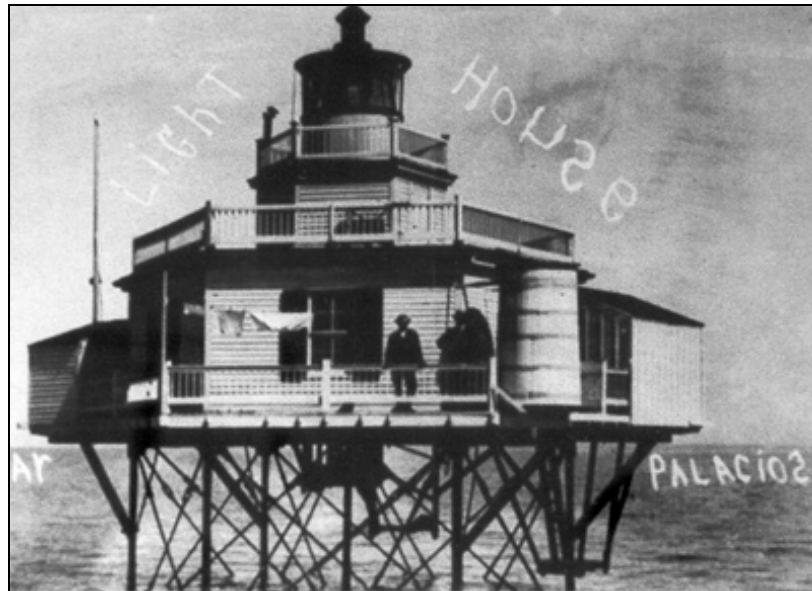
Figure 3-13. A photograph of the Halfmoon Reef Lighthouse made between 1902, when the lighthouse was reactivated, and 1911, when the second story deck was eliminated. A water cistern and two storage sheds or outhouses are built on the deck surrounding the main floor (Lighthousefriends.com 2009).
