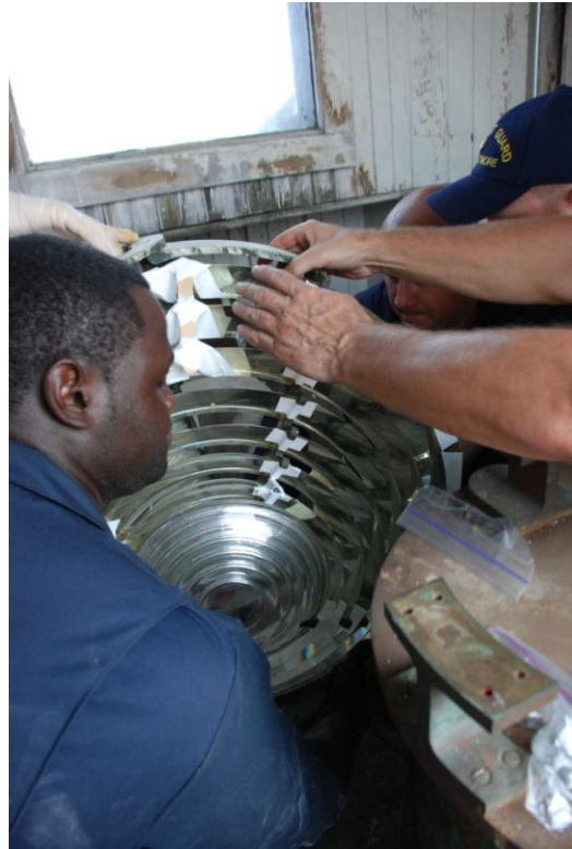
Removing the lens from the pedestal
