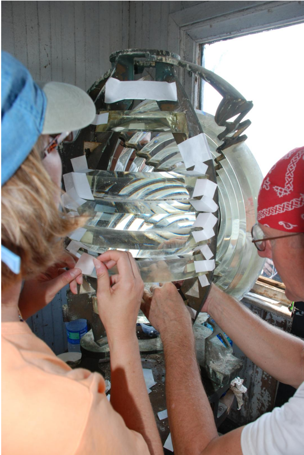
All of the prisms were stabilized with archival tape. Arlyn Danielson and Frank Blaha are placing tape on each prism.
