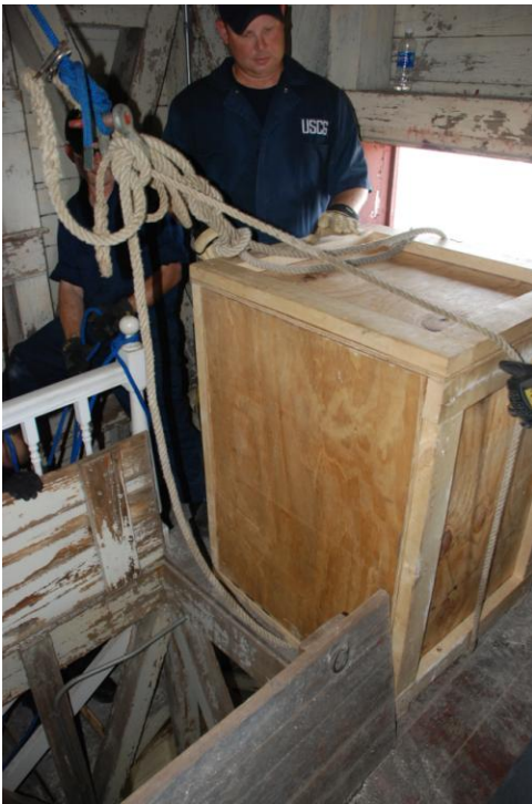
Once the lens was secured in the crate it was lowered down the shaft
