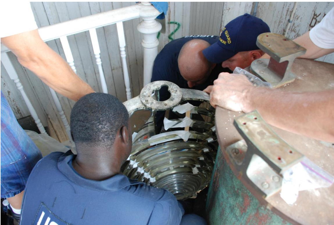
Removing the lens from the pedestal
