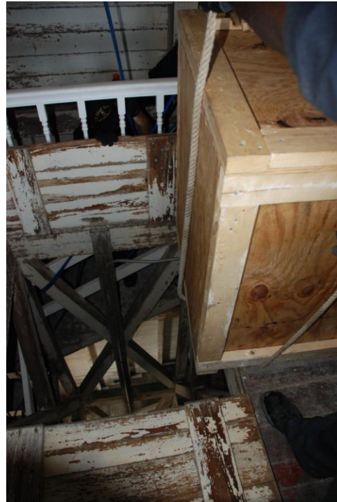
Once the lens was secured in the crate it was lowered down the shaft
