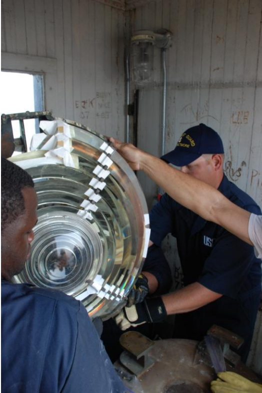
Removing the lens from the pedestal
