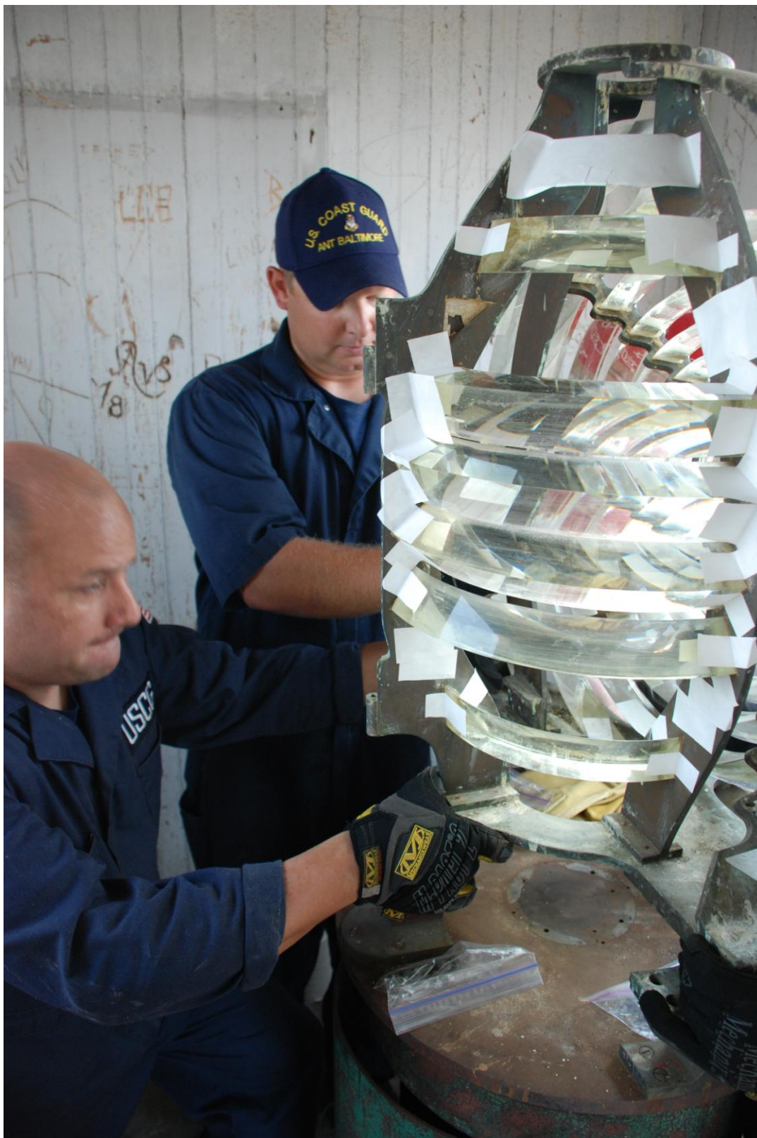
ANT Baltimore preparing to move the lens off of the pedestal
