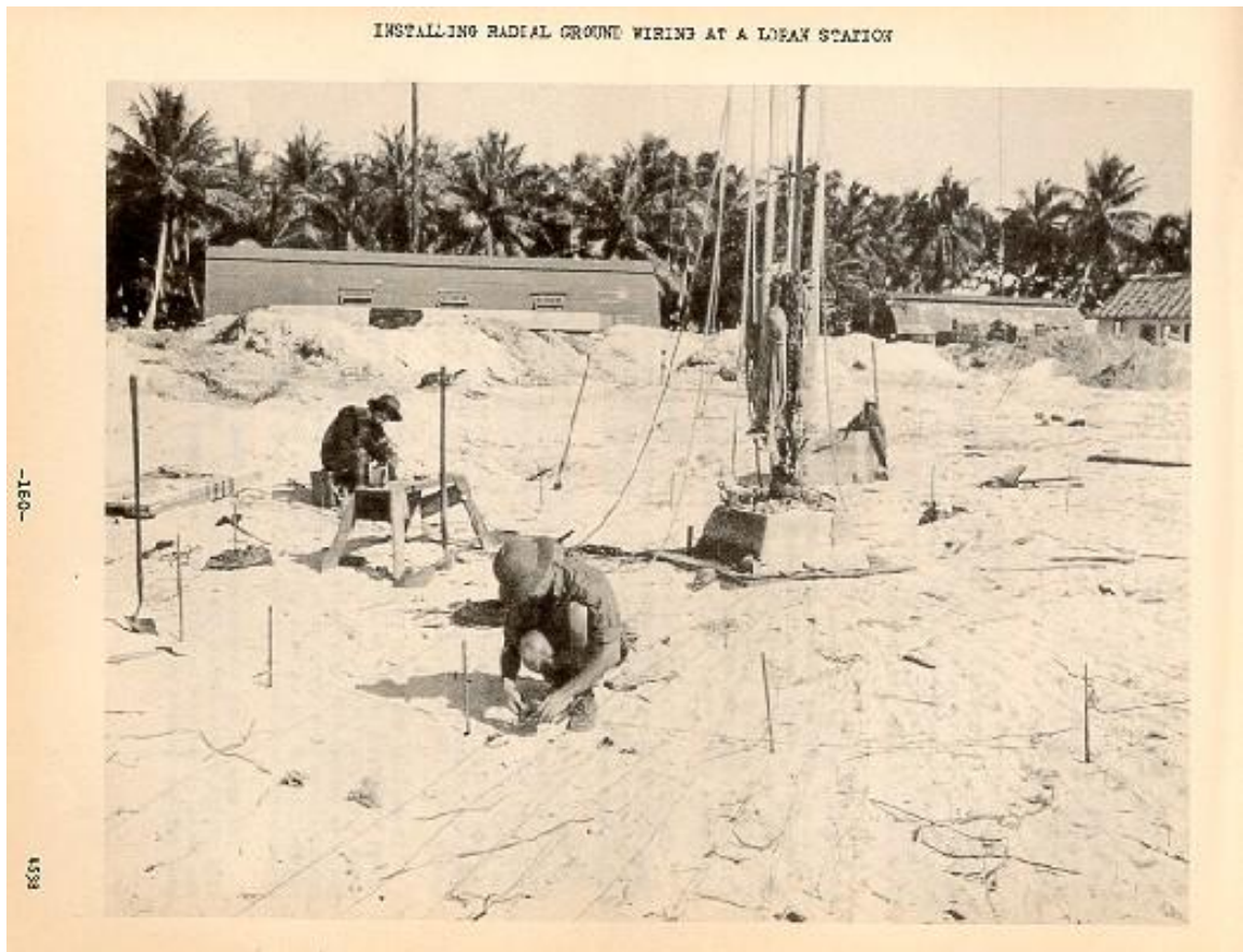
Image Caption: INSTALLING RADIAL GROUND WIRING AT A LORAN STATION
