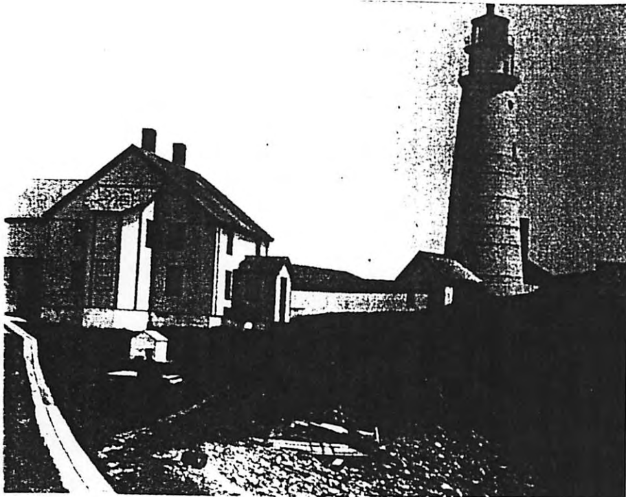
Assistant Keepers' House - around the turn of the century; note covered walkway from house to light tower [Photo #19; USCG]
