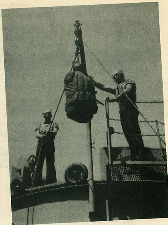
AFTER THE JACKET IS FITTED TO THE DUMMY COAST GUARDSMEN USE BLOCK AND TACKLE TO HOIST IT INTO POSITION ON TOP OF THE TANK
