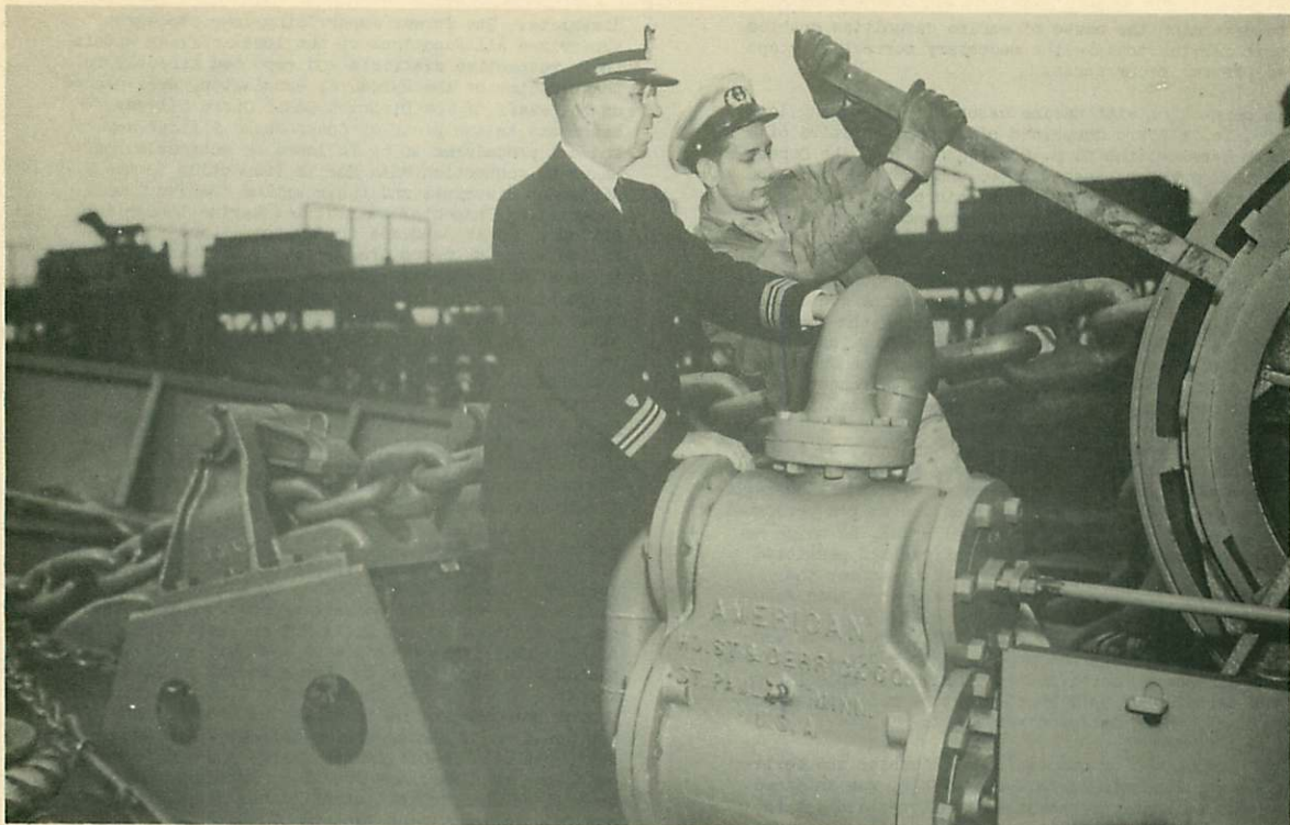
MEMBER OF THE COAST GUARD MARINE INSPECTION DIVISION EXAMINES THE ANCHOR WINDLASS, VITAL PART OF THE DECK MACHINERY
