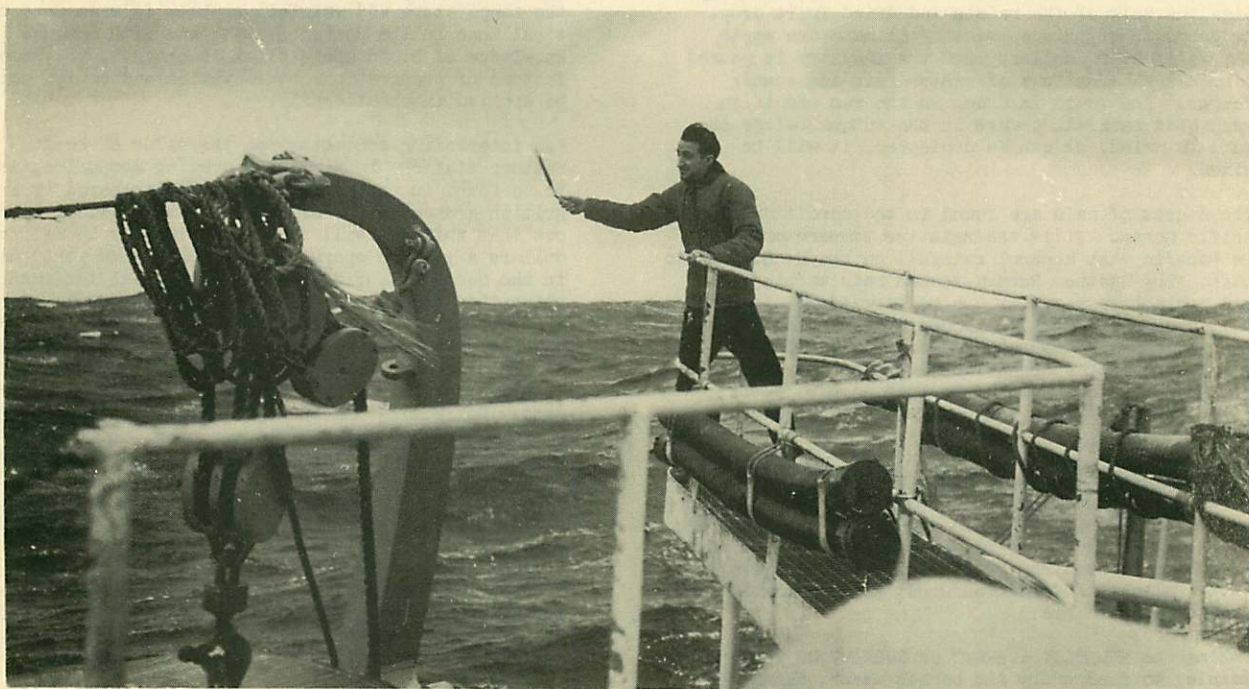
TWIRLING PSYCHROMETER TO OBTAIN SURFACE AIR TEMPERATURE AND HUMIDITY
