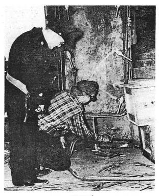
HOT WORK! STANDING FIRE WATCH WHEN WELDING AND CUTTING WERE BEING DONE WAS ONE OF MANY DUTIES PERFORMED BY TEMPORARY RESERVISTS
