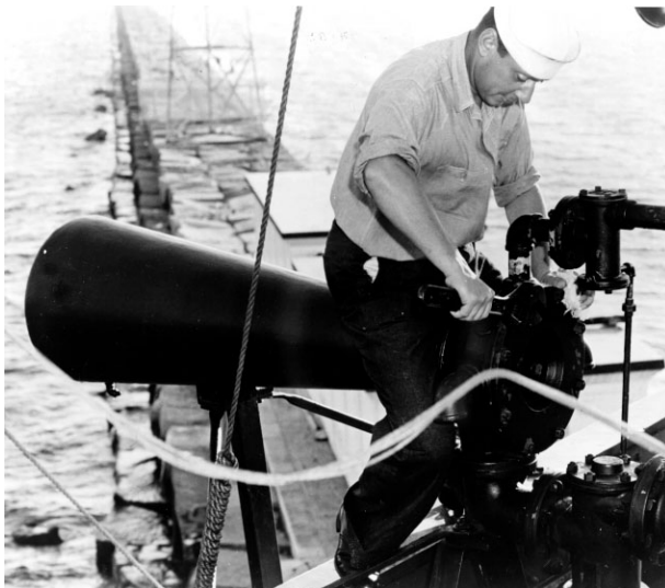
Working on the fog signal
