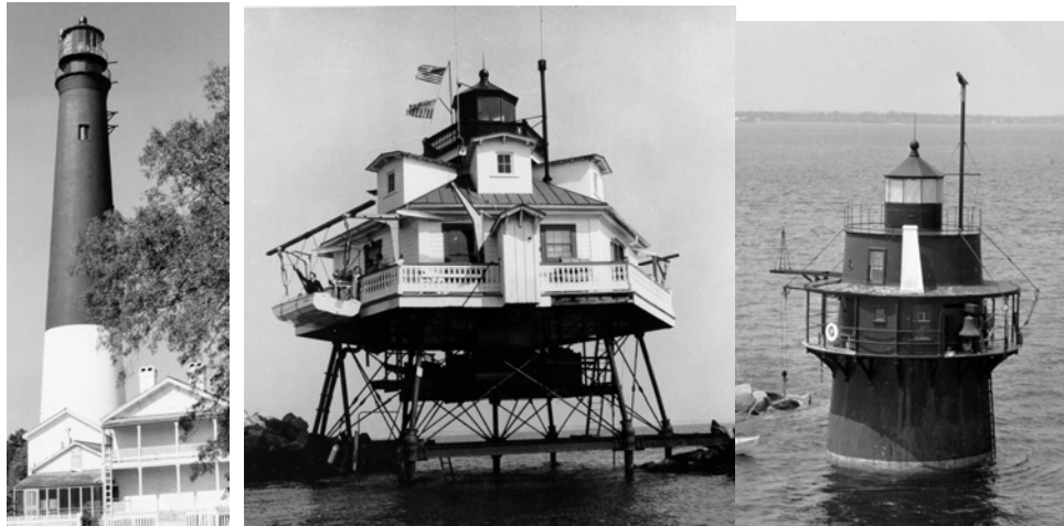
(L to R) Tall, conical light (Pensacola, FL); Screwpile light (Thomas Point, MD); Round caisson/sparkplug light (Duxbury, MA)
