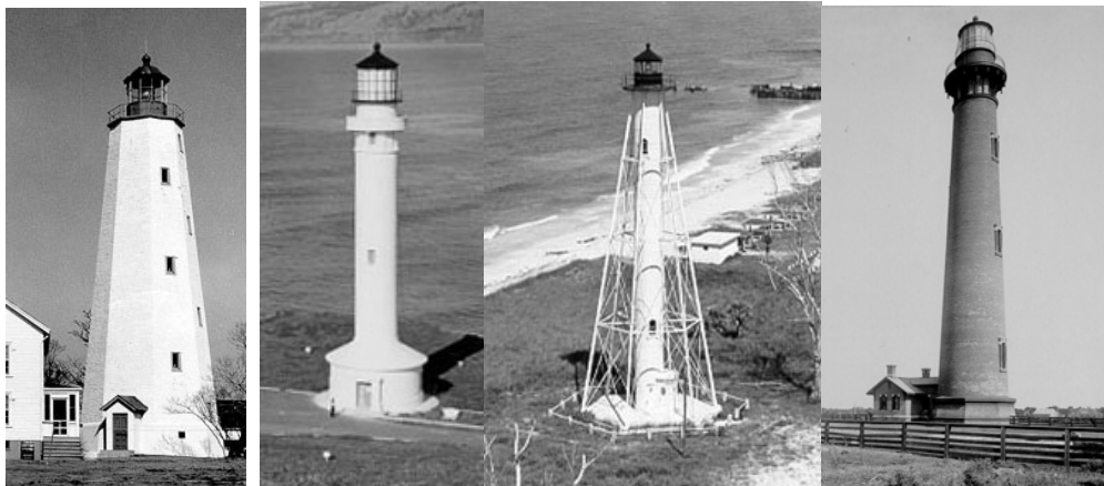
(L to R) Octagonal (8 sides) (Sandy Hook, NJ); Cylindrical (Point Arena, CA); Skeletal (Boca Grande, FL); Conical (Currituck, NC)
