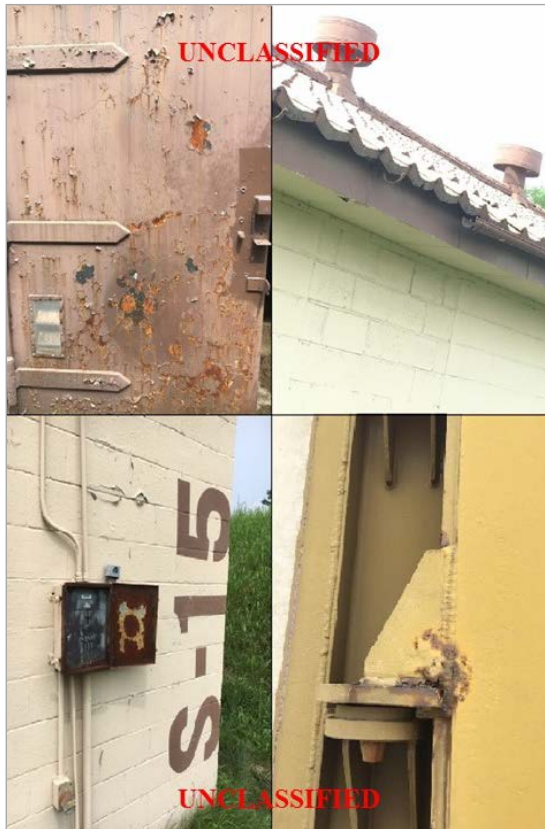
(U) Figure 4. Maintenance Deficiencies Observed: Rusted Door, Missing Gutter, Damaged Door Hinge, Rusted Breaker Box (Clockwise, From Top-Left)
