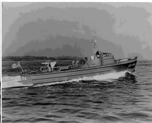
CG-457 circa 1942 mounts, 50-cal water cooled m.g. forward. CG-624 turning up the knots, mounts a 20-mm aft.
