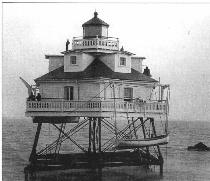
The first lighthouse at Sharps Island in the Chesapeake Bay was a screwpile design that was destroyed by drifting ice in 1881. It was replaced by a caisson tower (right) a few years later, but the annual assault by ice has caused the lighthouse to lean. Even so, it remains in service. Wikimedia Commons photo. Thomas Point Shoal Light (left) is the only screwpile lighthouse that remains in service on the bay. USLHS archives.
