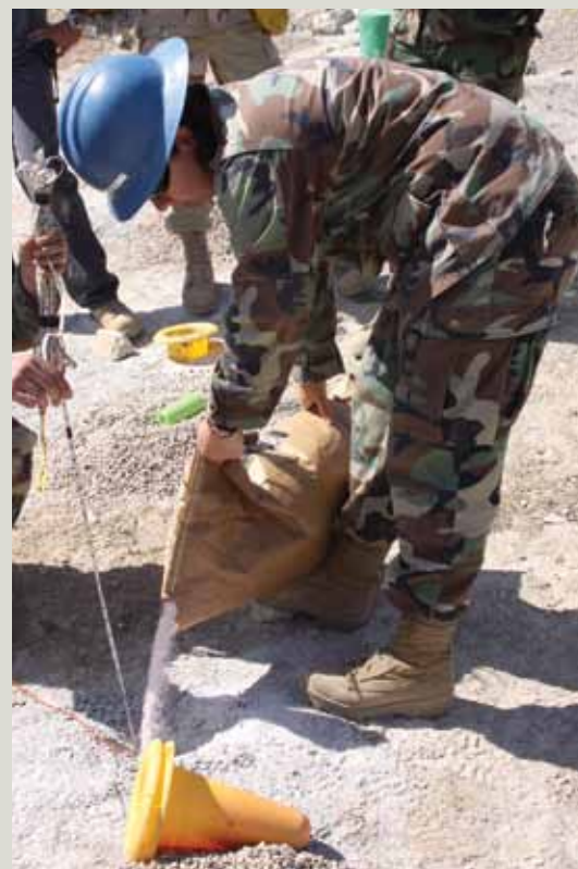
EO2(SCW) Bethany Pederson, NMCB 4, loads a bore hole with Ammonium Nitrate Fuel Oil (ANFO) in preparation for blasting during NCTC Blasting School, Naval Air Weapons Station, China Lake, Calif., April 29.
