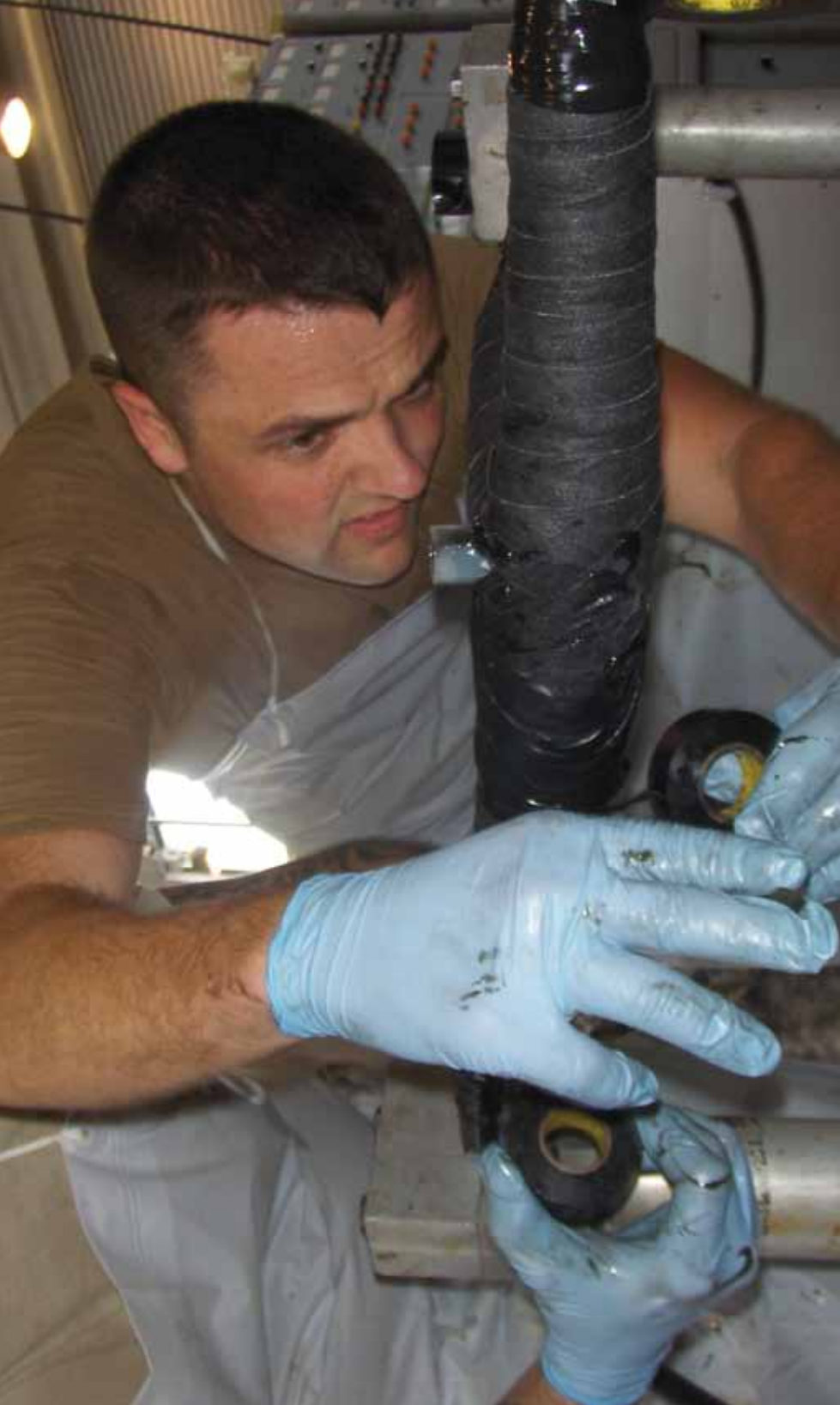
CM2(SCW) Luke Leifeste learns how to properly splice high-voltage cable during the Electrical Specialty Phase at Prime Power School, CSFE Detachment, Fort Belvoir, Va., in April. U.S. Navy photo
