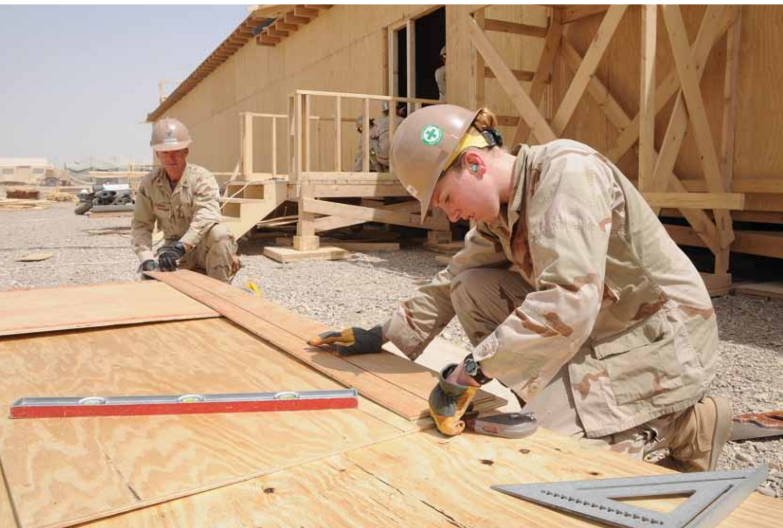
BUCN Leslie Stangler (foreground) and BU2 Jason Bowman, NMCB 5, mark a cut line for the staircase of a newly constructed Marine Expeditionary Battalion (MEB) building at Camp Leatherneck, Afghanistan, May 12.
