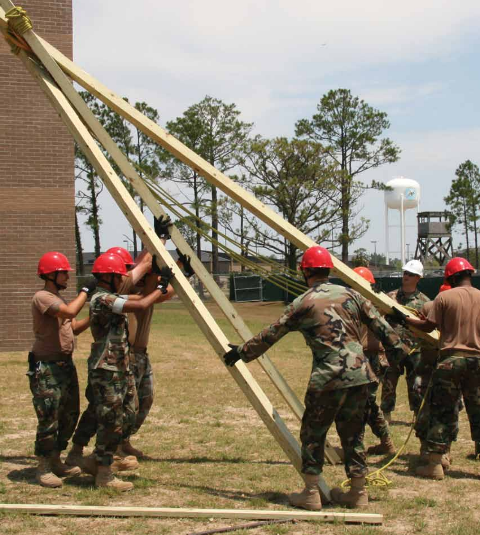
(Above) Disaster Recovery Team students erect a wooden casualty lifting as part of the final practical lab during Basic Rescue class, NCTC Gulfport, Miss., July 2009. U.S. Navy photo by Milt Williams
