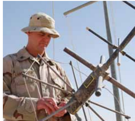
ET1 Bill Lancaster, NMCB 24, adjusts a UHF antenna, enabling more efficient communications at Al Asad Air Base, Iraq.
