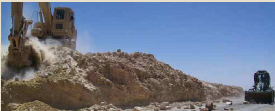
NMCB 24 equipment operators use an excavator and front-end loader to remove excess material from an embankment to repair a wash-out in Al Anbar province, Iraq, May 29.
