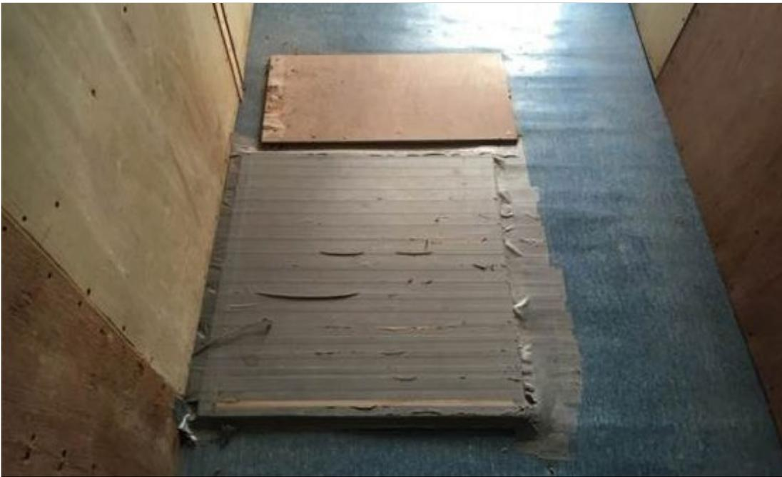
Figure 5. Temporary Patch for Holes in Housing Unit Floors
