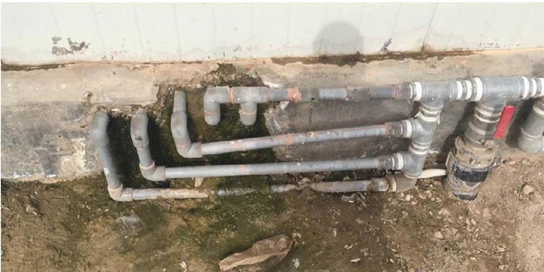
Figure 6. Water Leaks in the Delta Block
