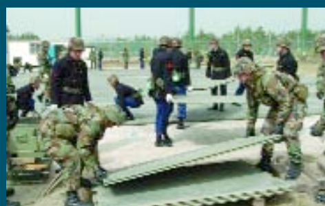
KOREA (Above, top to bottom) Seabees and Republic of Korea (ROK) sailors lay down M19 matting during a Rapid Runway Repair (RRR) exercise during Reception, Staging, Onward-movement and Integration (RSOI) 2006.
