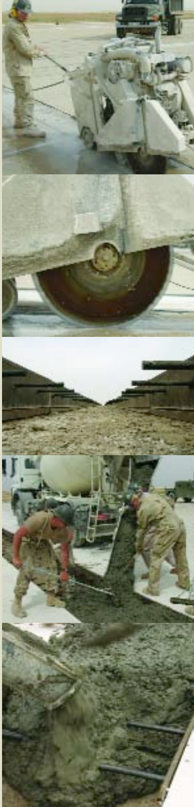
Seabees from NMCB 25 worked 24/7 repairing an Iraqi runway which had slowly deteriorated from constant extreme temperatures above 120 degrees Fahrenheit. Photos above depict various phases of runway repair and reconstruction. U.S. Navy Photos
