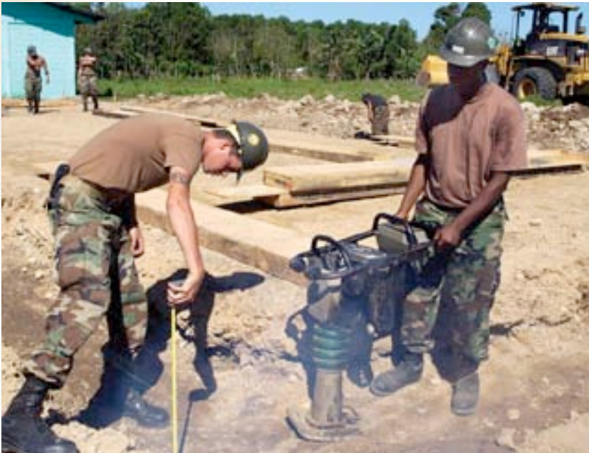
Builder Constructionman Mike Veroneau, left, measures the trench depth as Construction Electrician 3 rd Class Justin Nice operates the wacky packer NMCB 7 conducted a humanitarian project in support of New Horizons, a $6 million joint U.S.-Honduras military humanitarian exercise. New Horizons provided new schools at El Pino, Los Girasoles, Gonzalo River and El Cacao, with one maternity clinic at Jutiapa. In addition, 14 health clinics were offered from Mosquito Coast to San Pedro Sula.
