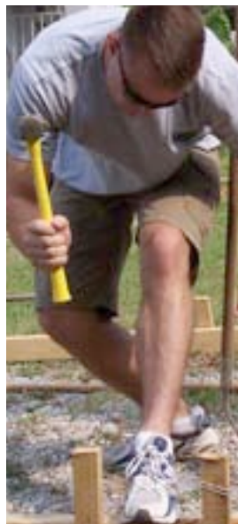
Construction Equipmentman 1 st Class Michael Copponi drives in a support stake for the sidewalk frame during a community relations project sponsored by NMCB 74 First Class Petty Officer Association (FCPOA).
