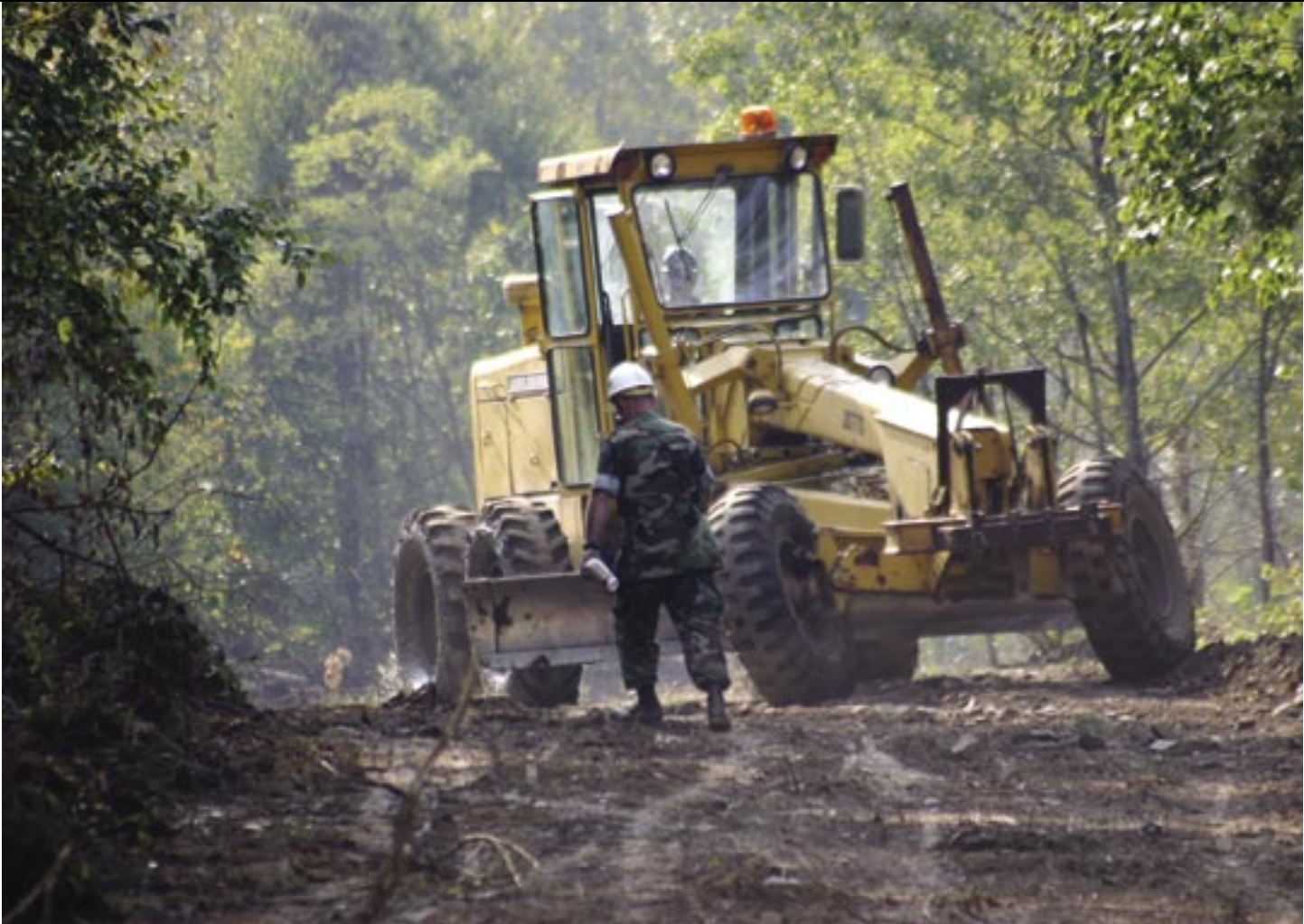
EOC(SCW) Martin O'Horo gives instruction on the use of a grader to E03 Robert Maslyar. As with many Seabee training projects, the road-cutting job prepared NMCB 21 for an upcoming field exercise and provided hands-on training with large-vehicle operations. The road construction facilitated transportation of boats to a flooded strip mine pit police investigators wanted to search in order to recover evidence crucial to their case.
