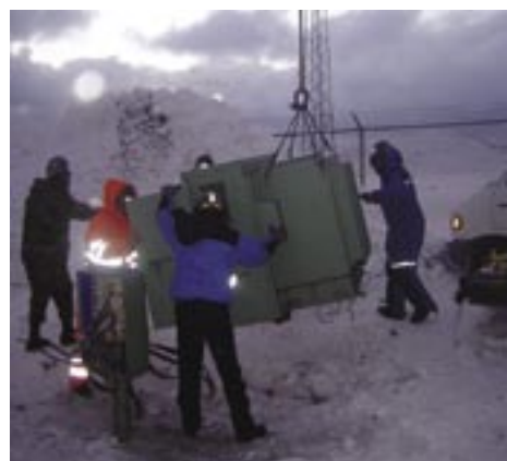
Broken transformer is removed
