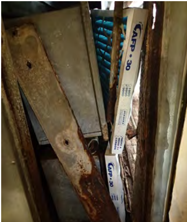
Figure 9. Significantly damaged HVAC filter bank found in NS Mayport unaccompanied housing building 2105. (Deficiency No. MAY-EN-150302-007) Source: DoD OIG
