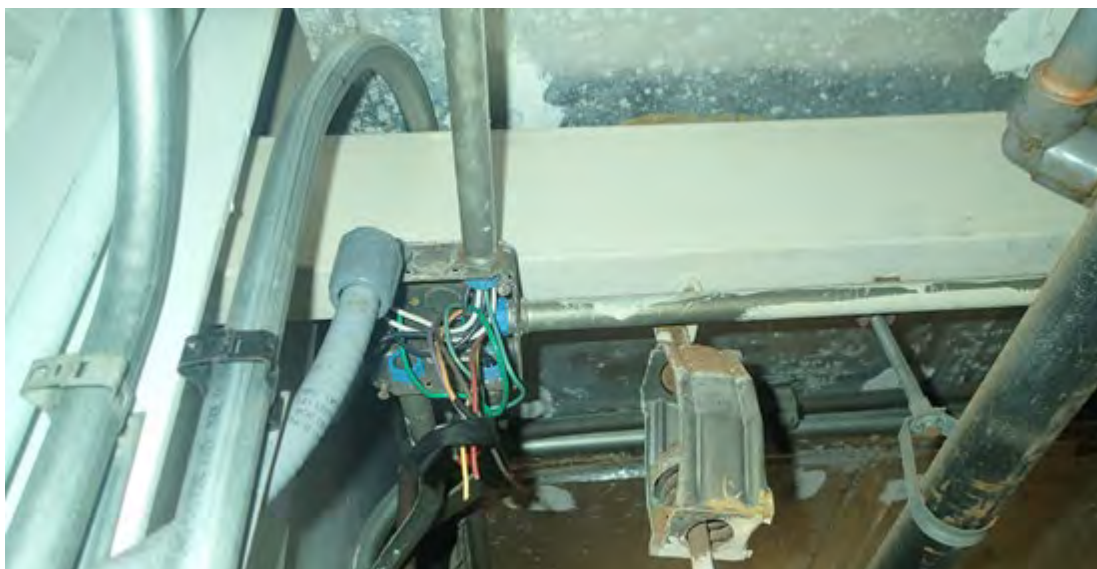
Figure 8. Exposed wiring in a mechanical room of NS Mayport unaccompanied housing building 1587. (Deficiency No. MAY-EL-150302-022) Source: DoD OIG
