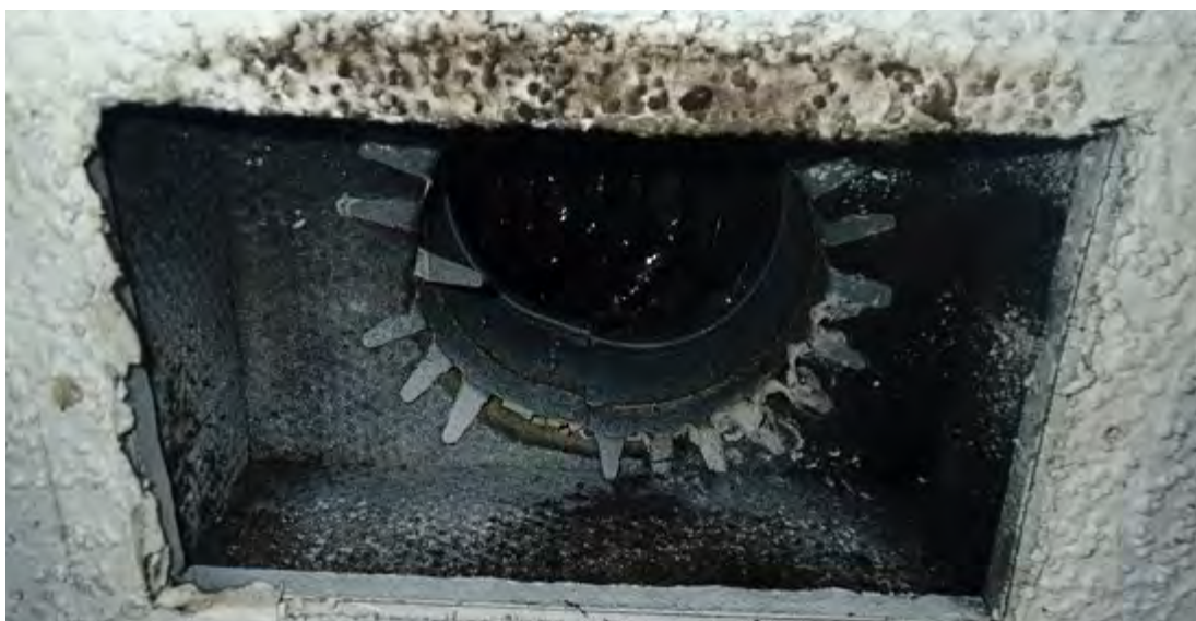
Figure 5. Visible mold and excessively dirty HVAC ductwork in Patrick AFB River's Edge housing unit. (Deficiency No. PAT-EN-150223-015) Source: DoD OIG
