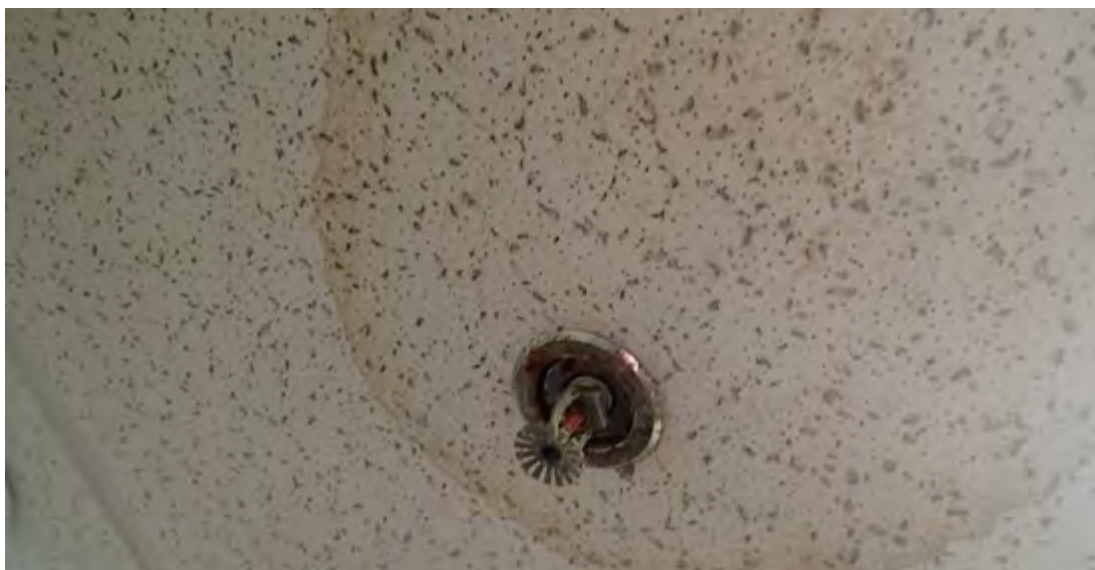
Figure 3. Severely corroded fire suppression sprinkler heads in Patrick AFB's unaccompanied housing building 505. (Deficiency No. PAT-FP-150223-02) Source: DoD OIG
