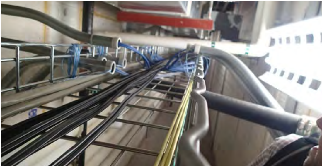
Figure 11. Combustible and non-plenum-rated materials present in Fort Gordon's TBUP-renovated building utility corridors used as airways. (Deficiency No. FGN-FP-150309-053) Source: DoD OIG
