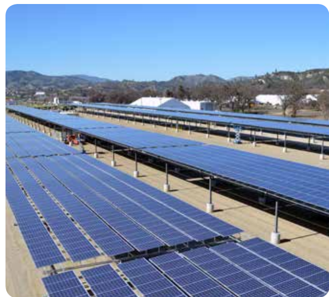
Fort Hunter Liggett Solar Photovoltaic Energy Conservation Investment Program project. (Photo by John R Prettyman)
