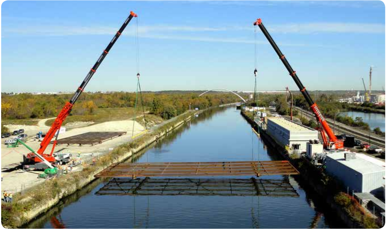
Underwater structures, known as parasitics, being placed into the Chicago Sanitary and Ship Canal by the barriers to the areas designed for fish deterrence. (U.S. Army Photo by Sarah Gross/Released)
