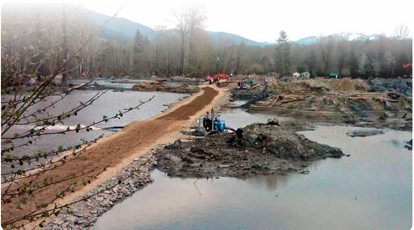
The U.S. Army Corps of Engineers, Seattle District, has nearly completed construction of the temporary berm within the SR530 slide area. (Photo courtesy of U.S. Army Corps of Engineers)
