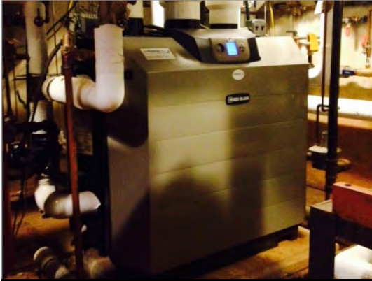
Figure 1. ECM 1 Boiler in Building 2784 Source: DoD OIG
