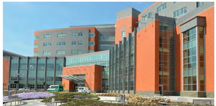
Figure 1. Entrance for Fort Belvoir Community Hospital Source: www.fbch.capmed.mil
