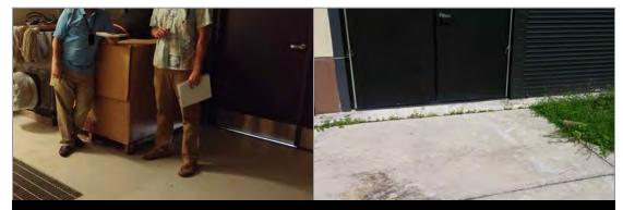
Figure 2. Visible Gap Under Hazardous Waste Storage Room Door. Exterior View Shows Close Proximity to Surrounding Environment.
