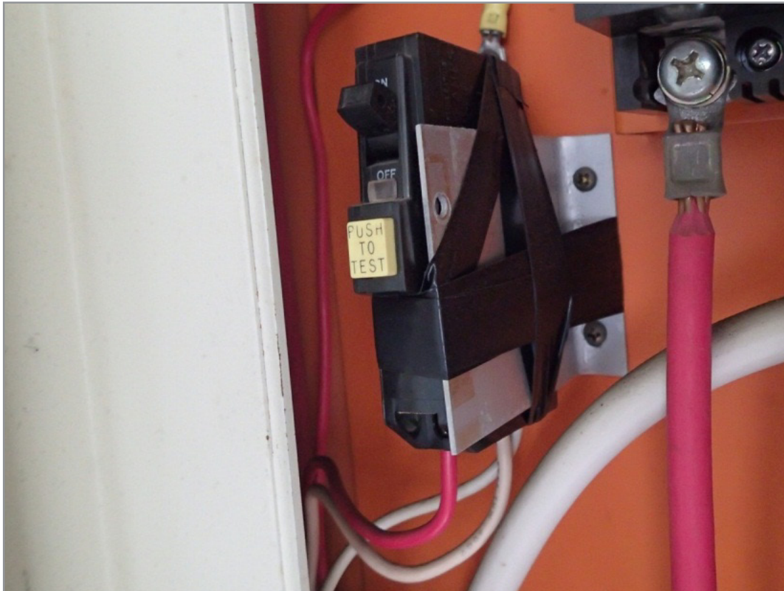
Figure 6. GFCI improperly secured in electrical panel (Deficiency No. YOK-EL-130925-005) Source: DoD OIG
