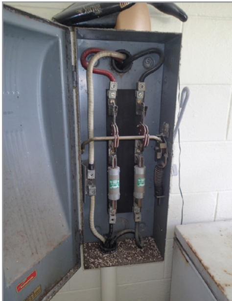
Figure 9. No earth grounding electrode conductor in service panel for single family house (Deficiency No. FOS-EL-131104-057) Source: DoD OIG
