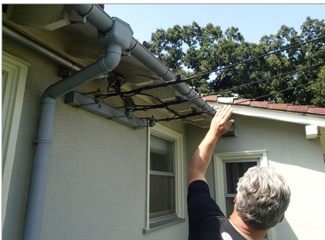
Figure 5. Example of low-hanging electrical service drops at housing units (Deficiency No. ZAM-EL-130923-012) Source: DoD OIG
