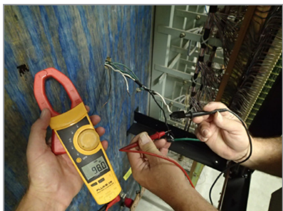
Figure 3. Live wires hanging out of wall without proper enclosure protecting from accidental contact (Deficiency No. ATS-EL-130917-018) Source: DoD OIG
