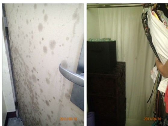
Figure 4. Left: Mold blooms inside barracks (Deficiency No. ATS-EN-130917-009A) Right: Warped paint from moisture/condensation inside single family housing unit (Deficiency No. ATS-EN-130917-008A) Source: DoD OIG
