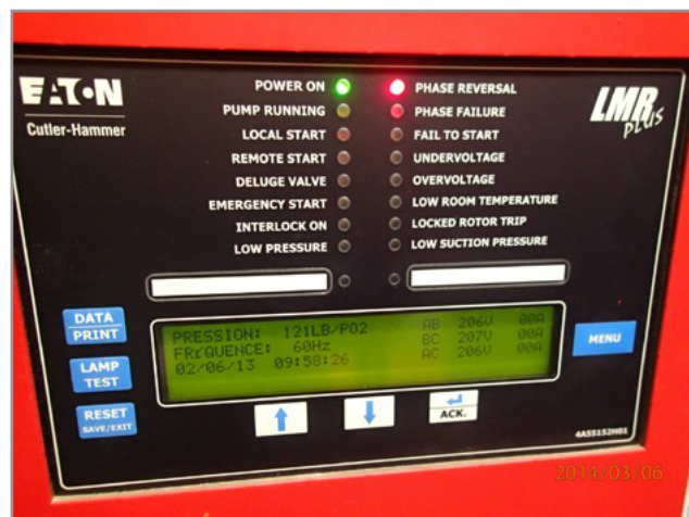
Figure 7. Fire pump controller electrical phase reversal fault rendering the fire pump and the sprinkler system completely out of service (Deficiency No. IWA-FP-140303-103) Source: DoD OIG
