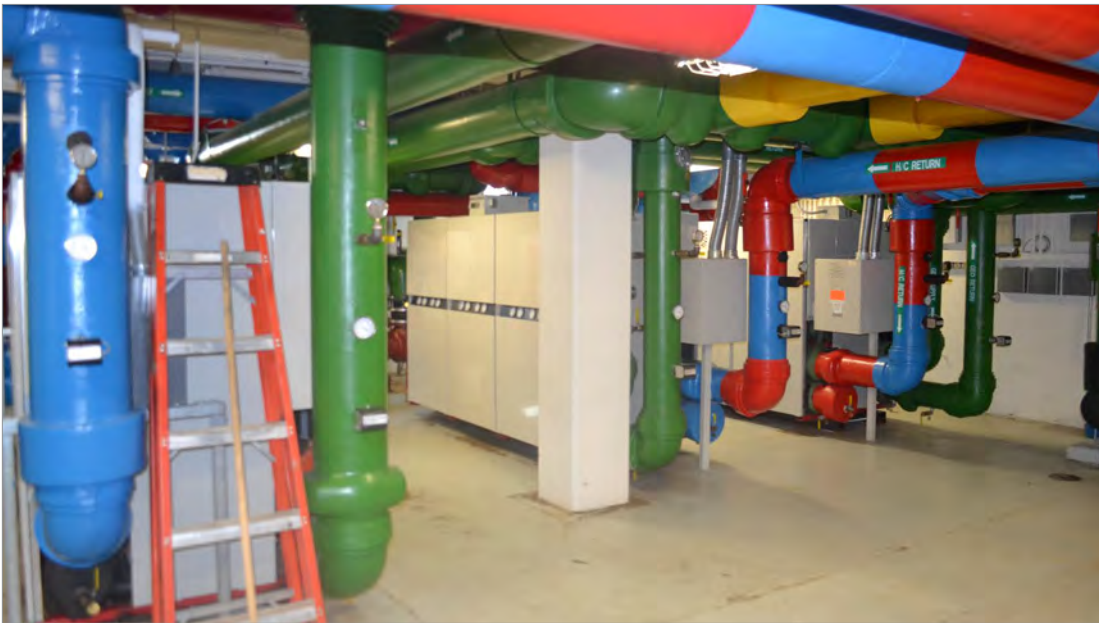
Figure 3. Geothermal Heating and Cooling Upgrades Source: DOD OIG
