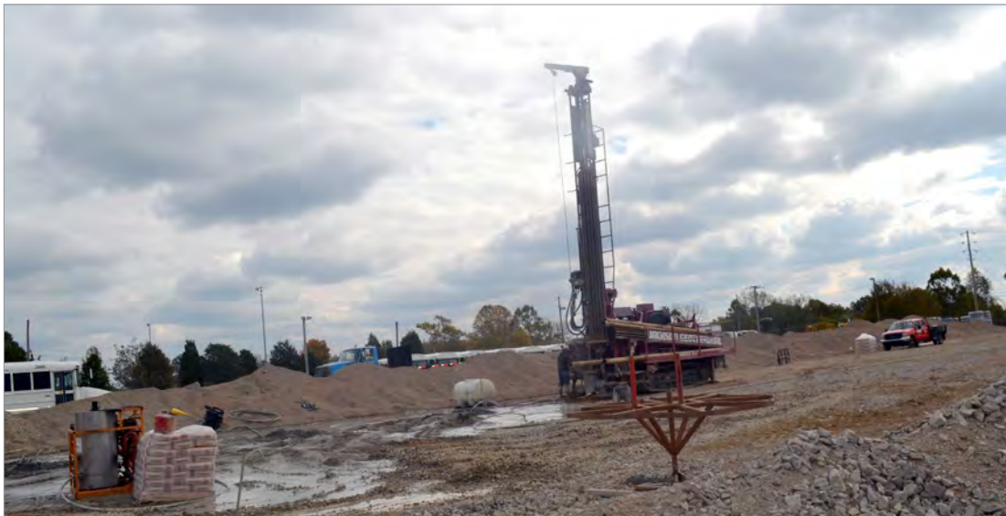
Figure 2. Ongoing Construction of Underground Loop of Pipes Source: DOD OIG
