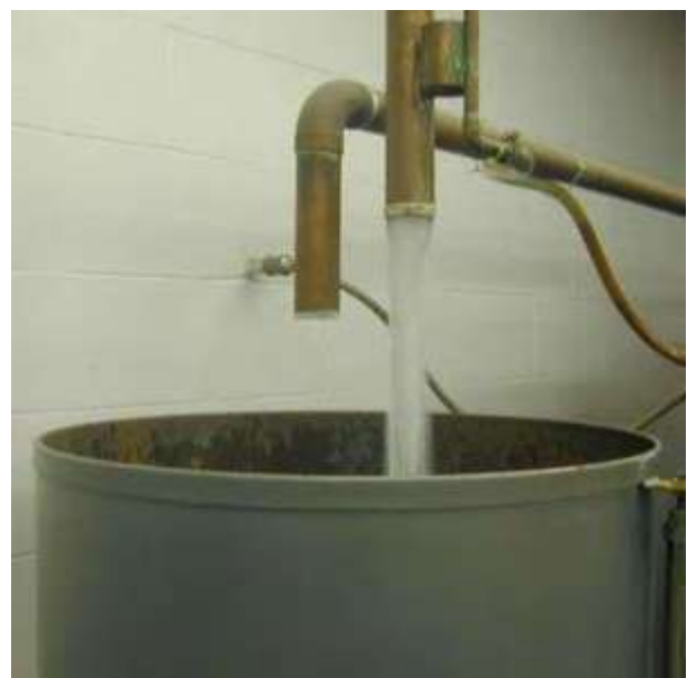
Figure 14-15 — Air gap. 14-37
