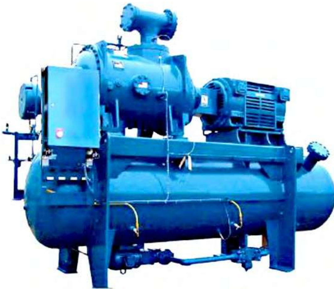
Figure 13-14 — Rotary screw compressor unit.
