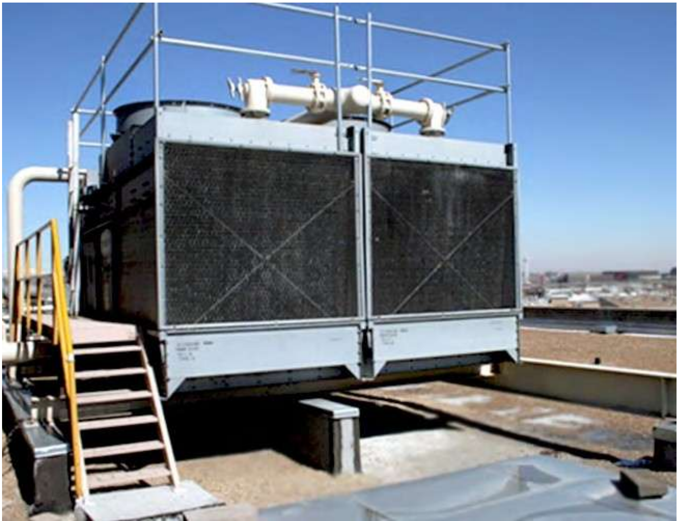
Figure 13-22 — Paralleled package towers.
