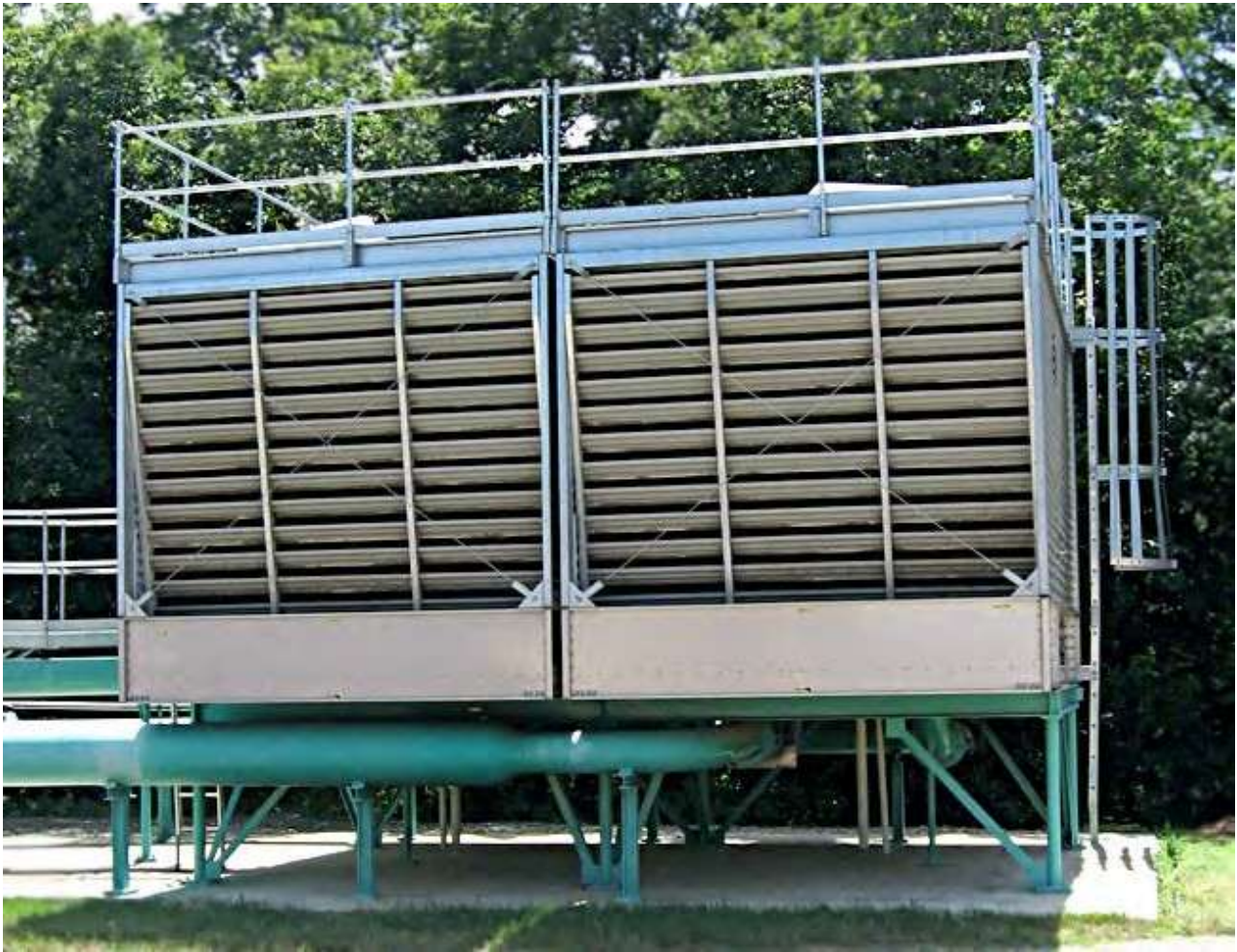
Figure 13-21 — Package tower with a remote, variable speed pump.
