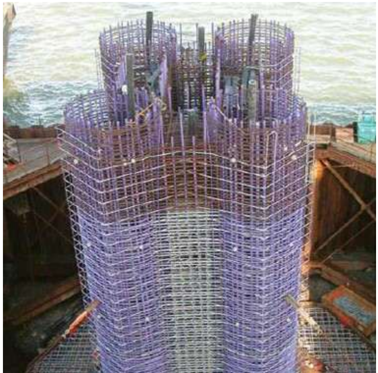
Figure 19-2 — Complex use of reinforcement bars.
