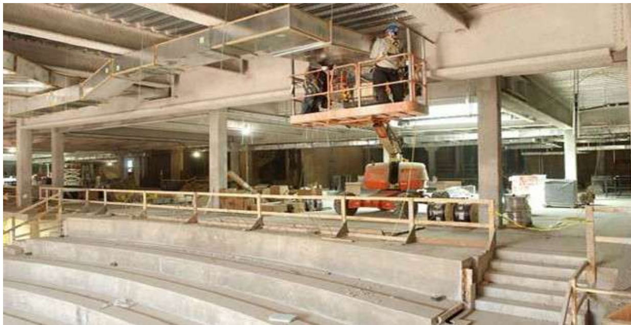
Figure 13-103 — Duct installed to a built up steel roof.
