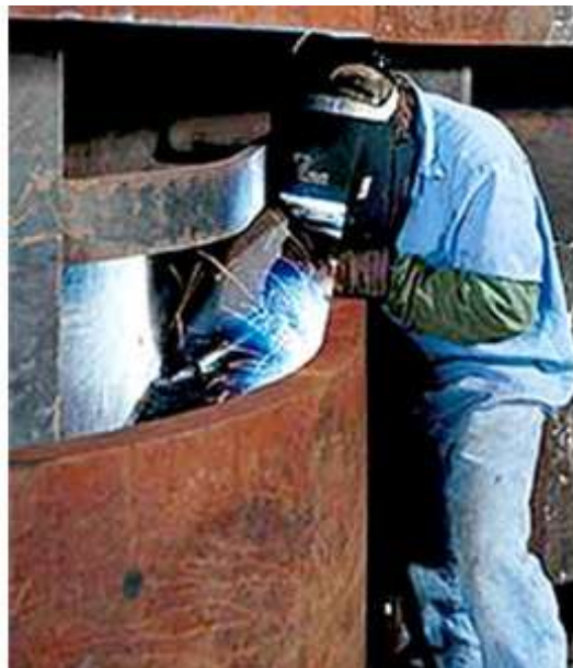
Figure 11-27 — Flux cored arc welding of structures.
