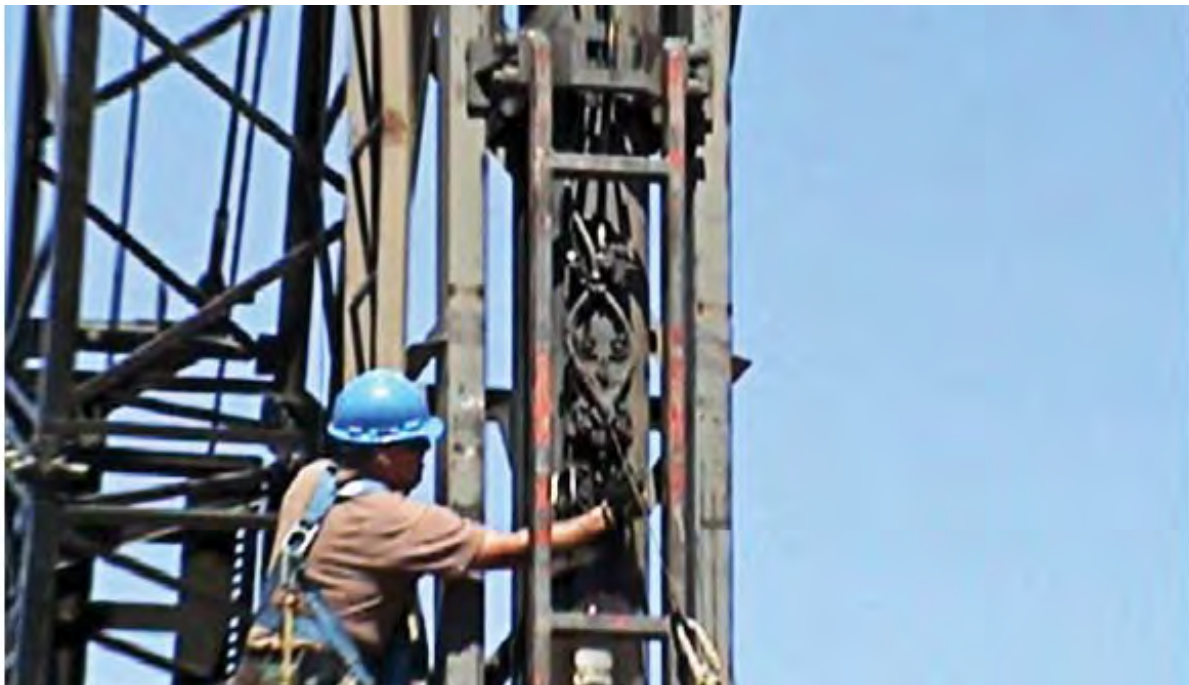
Figure 21-58 –Increasing fuel delivery (hammer in operating position).
