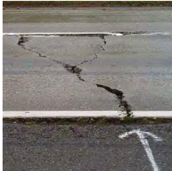
Figure 23-9 – Edge cracks.
