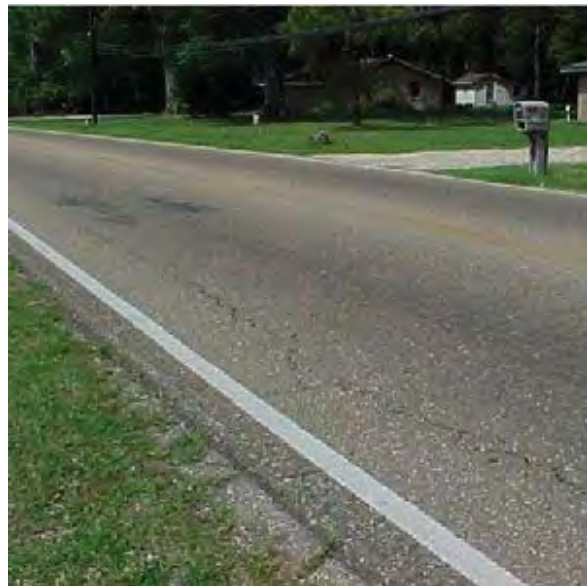
Figure 23-13 – Shrinkage cracks.
