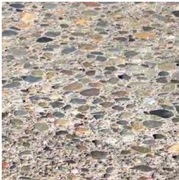
Figure 23-18 – Polished aggregate in pavement surface.
