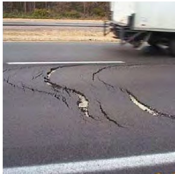
Figure 23-14 – Slippage cracks.
