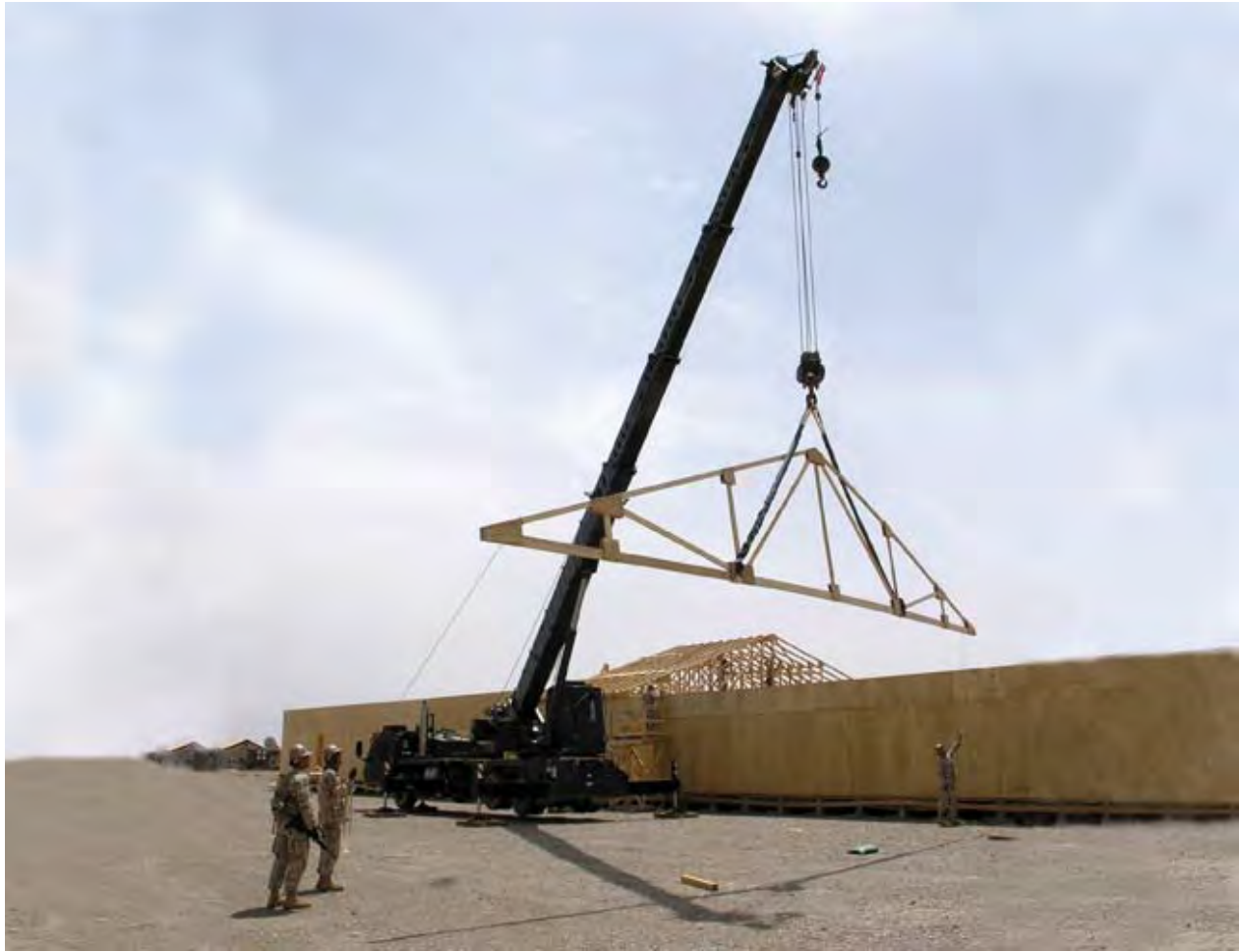
Figure 21-23 – Telescopic boom sections.
