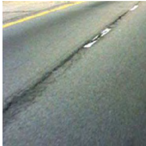
Figure 23-11 – Lane joint cracks.
