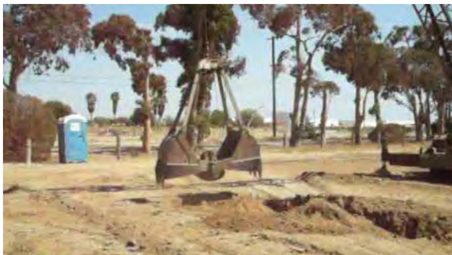
Figure 21-32 – Clamshell in operation.
