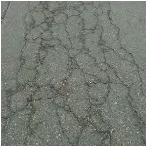
Figure 23-8 – Alligator cracks.
