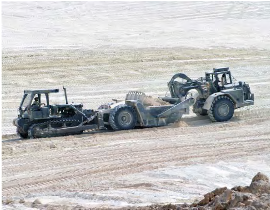
Figure 18-2 – Push cat pushing scraper.
