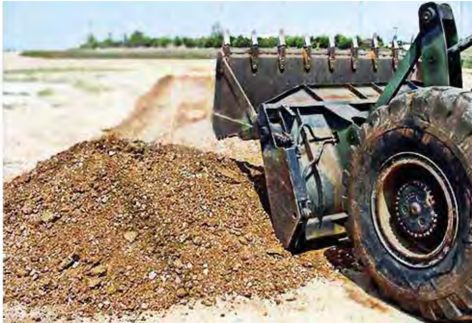
Figure 13-30 – Backfilling a trench.
