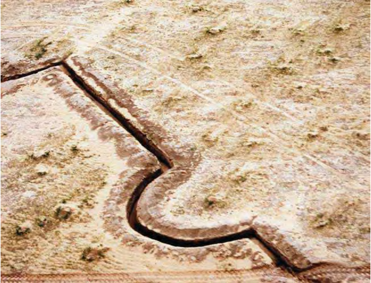
Figure 16-1 – Trench dug by ditcher.
