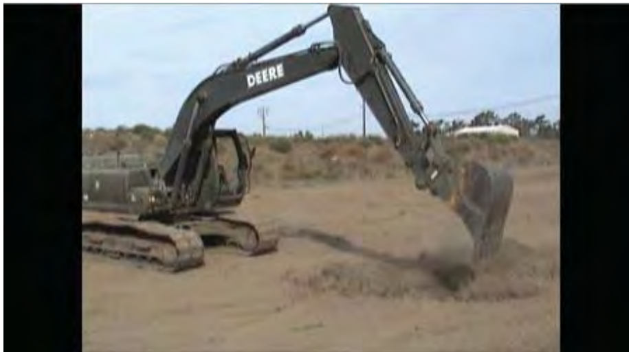
Figure 15-17 – Filling the bucket.
