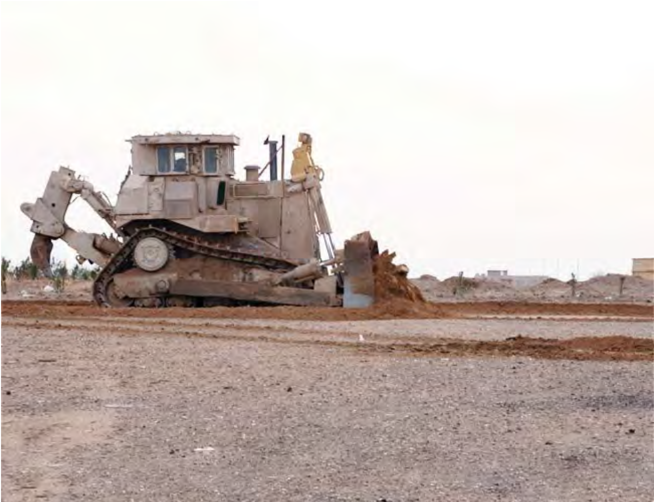
Figure 19-2 – High track dozer.
