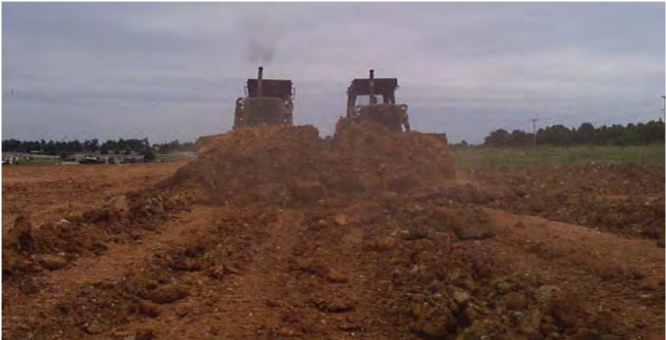
Figure 19-21 –Side-by-side dozing.
