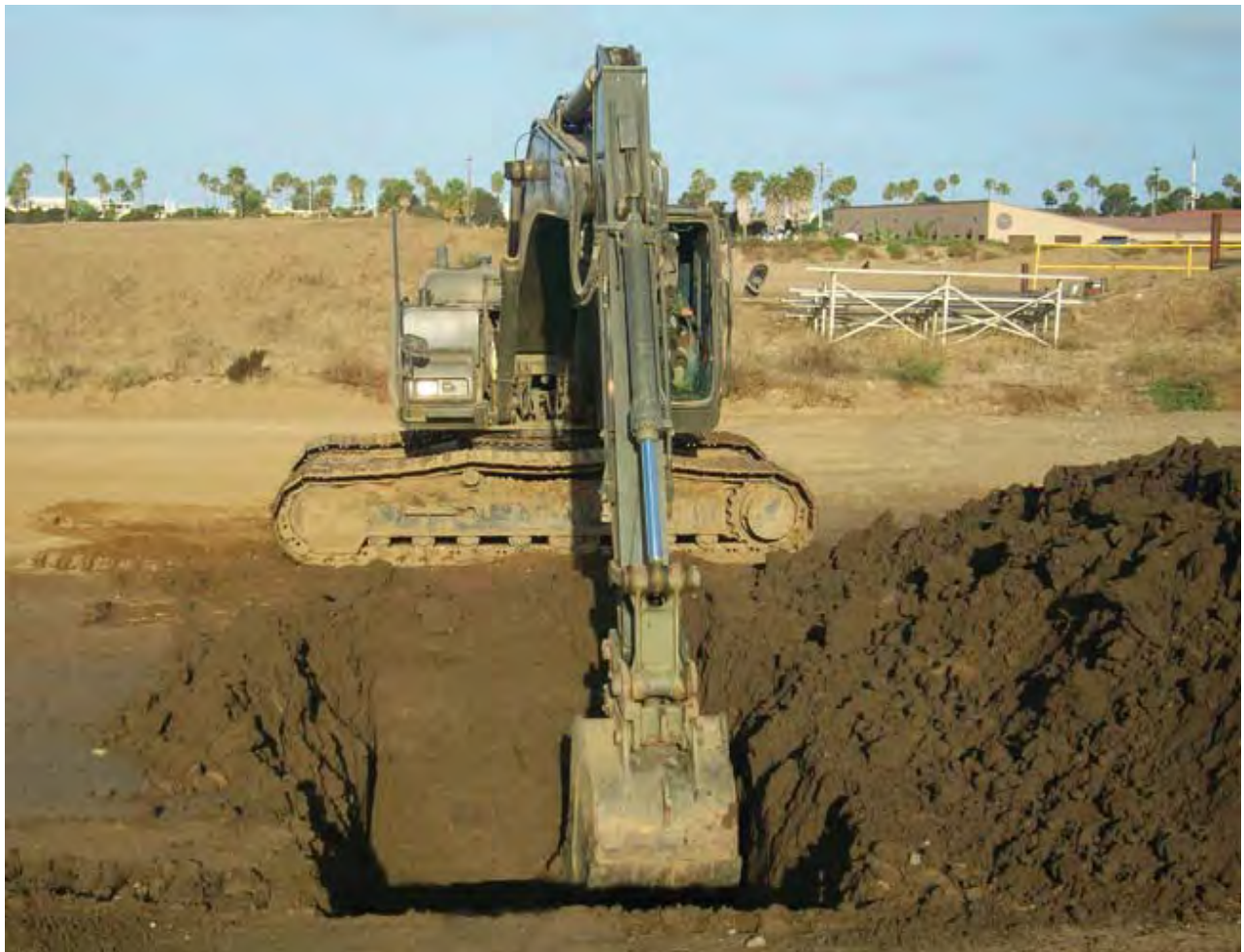
Figure 15-18 – Parallel position at trench.
