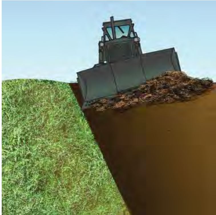
Figure 19-27 – Angle blade ditch cut.
