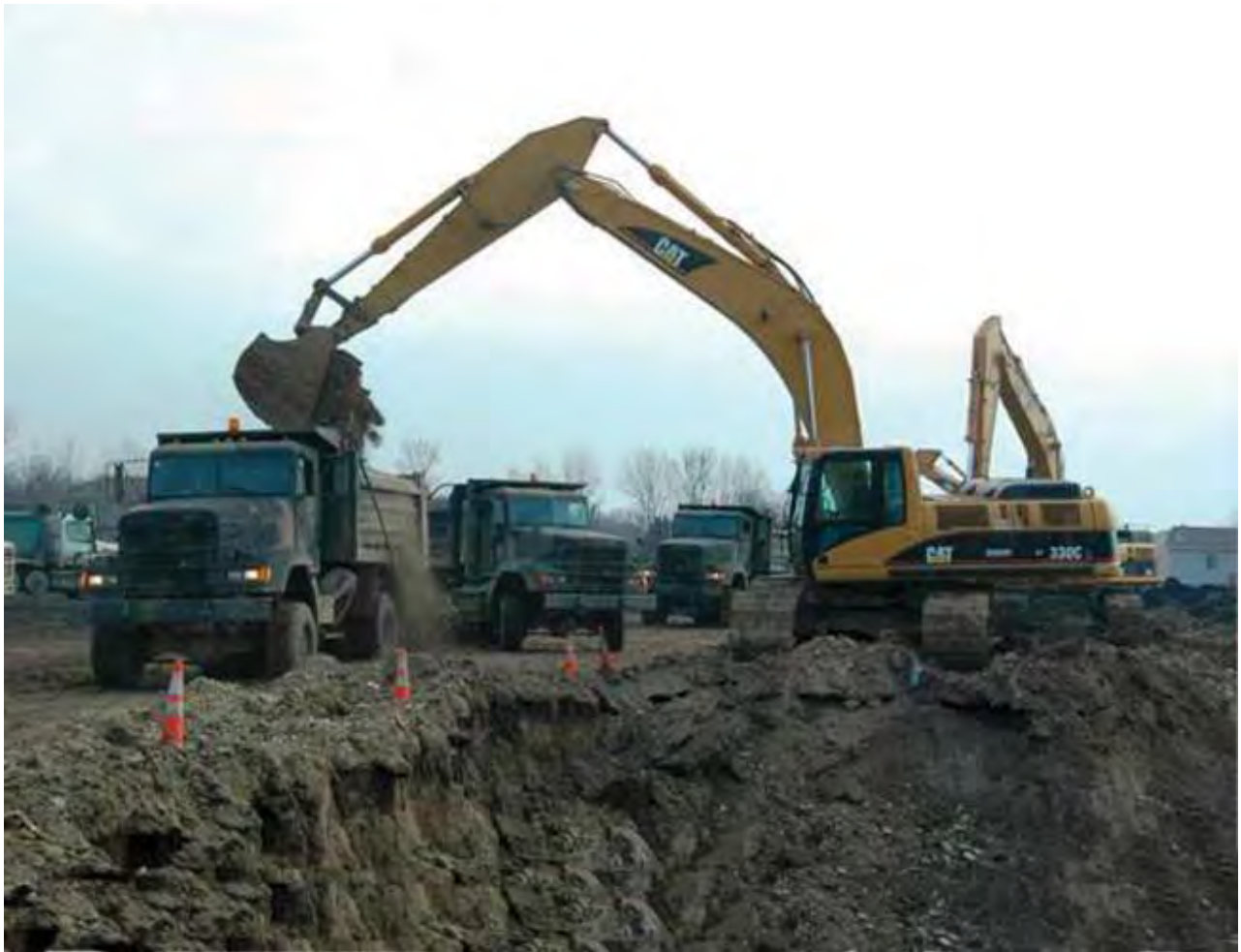
Figure 15-2 – Loading a dump truck.
