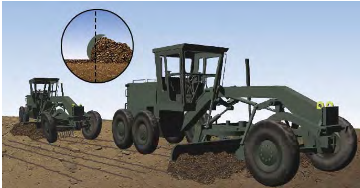
Figure 17-28 – Blade-mixing operations.
