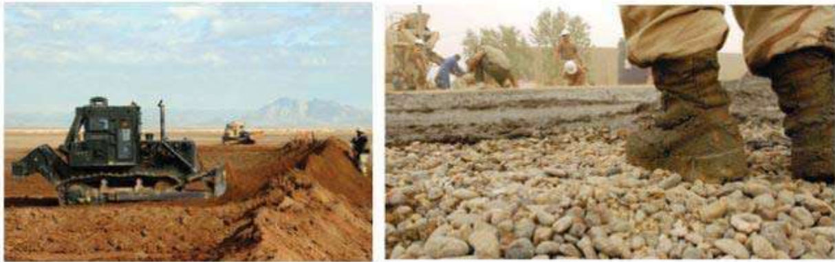
Figure 16-58 - Materials testing applies to soils, aggregate, and concrete.
