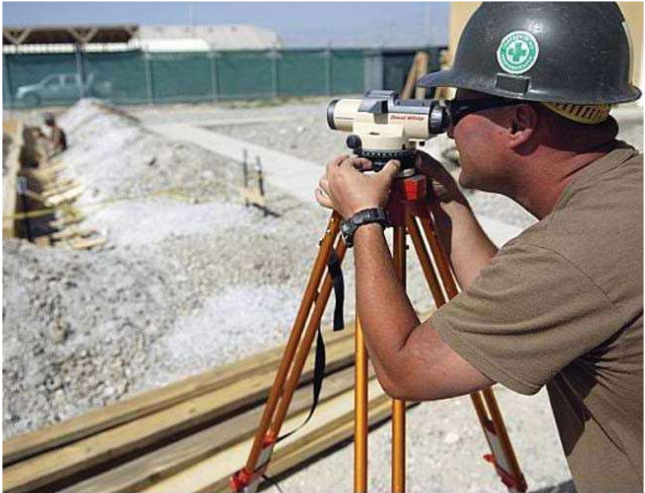
Figure 17-5 – Example of self-leveling level.
