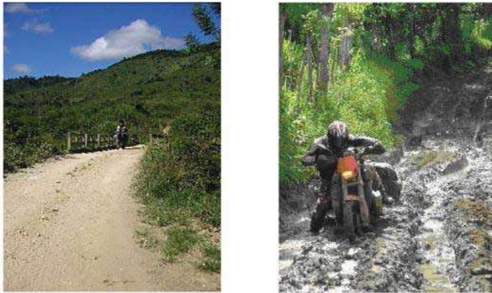
Figure 16-5 - Examples of clay road under dry and wet conditions.
