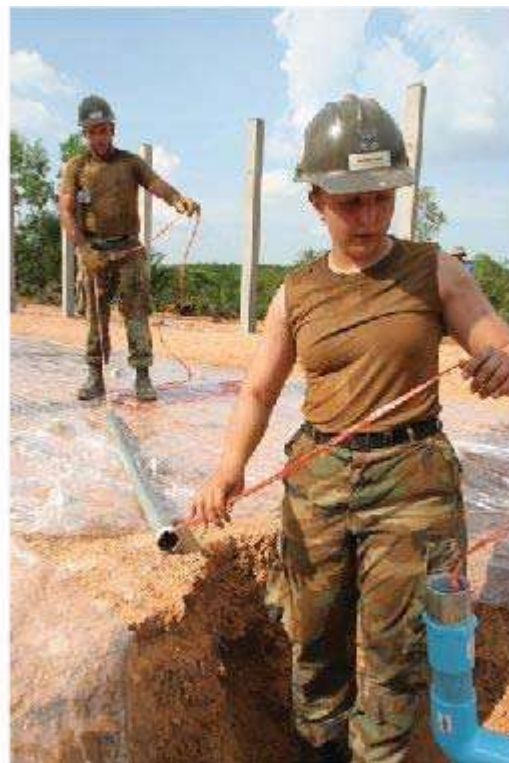
Figure 10-23 — Seabees installing PVC conduit.
