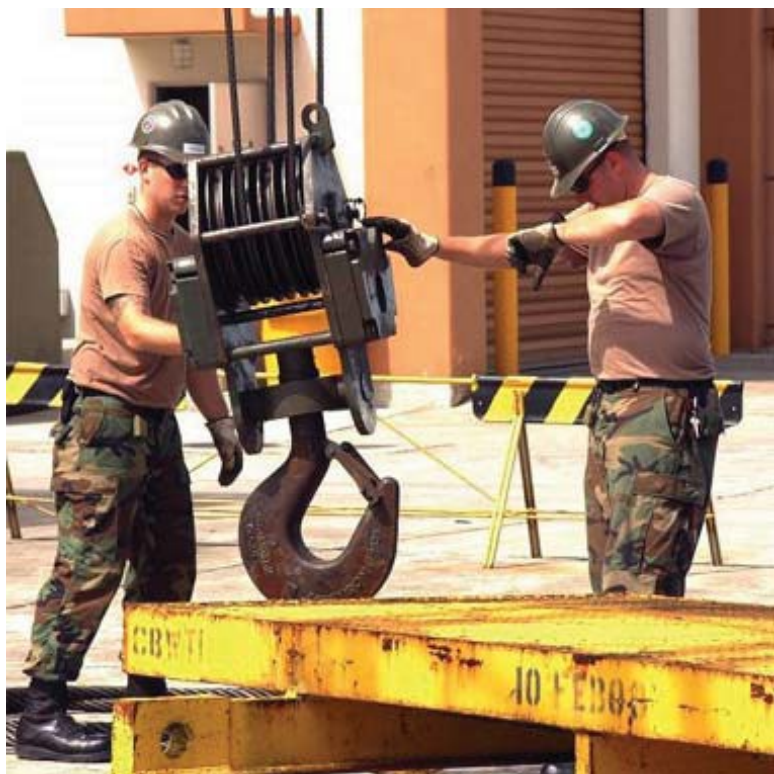
Figure 3-17 - Construction mechanics hooking the hoist of the crane to a calibrating weight to certify the crane.
