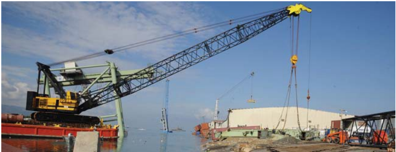
Figure 3-6 – Example of Category 1 cranes.
