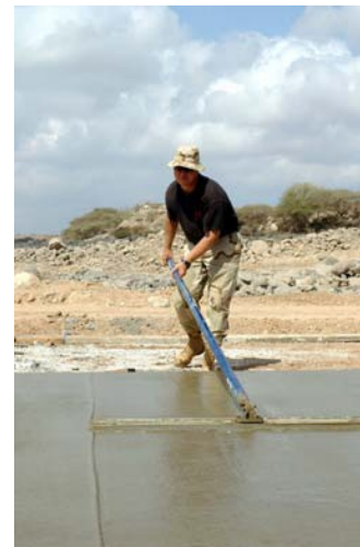
Figure 6-71 – Long handled float in use.
