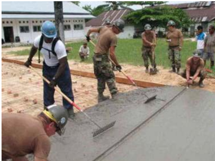
Figure 6-65 – Screeding operation.
