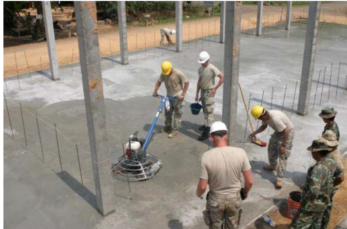
Figure 6-76 – Mechanical troweling machine.
