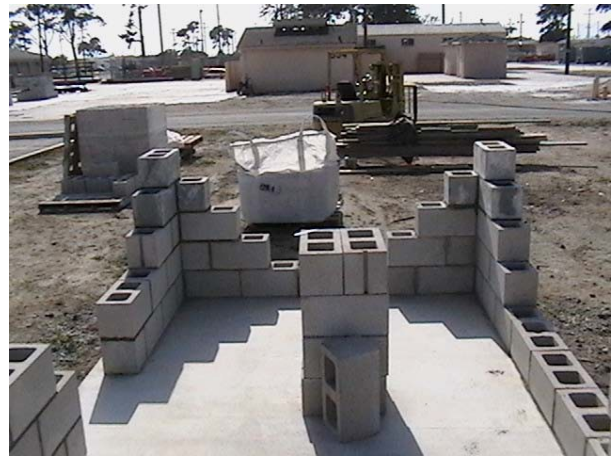
Figure 8-19 – Completed corner leads.
