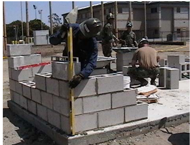
Figure 8-22 – Checking for plumb.
