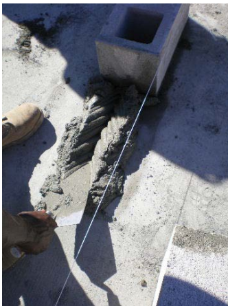
Figure 8-14 – Spreading and furrowing mortar bed.
