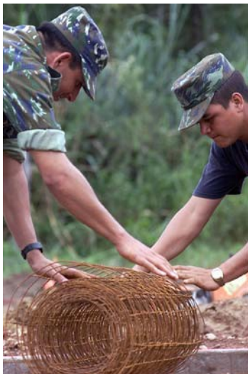
Figure 6-51 – Welded wire mesh fabric.
