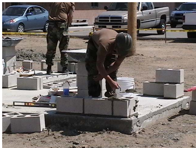
Figure 8-15 – Positioning and aligning corner block.
