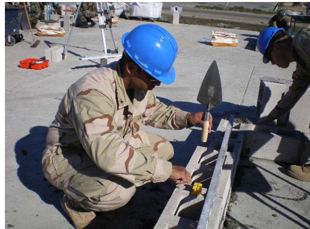
Figure 8-17 – Leveling block for a wall.
