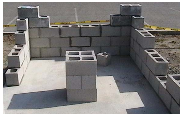
Figure 8-25 – Filling in the wall between corners.
