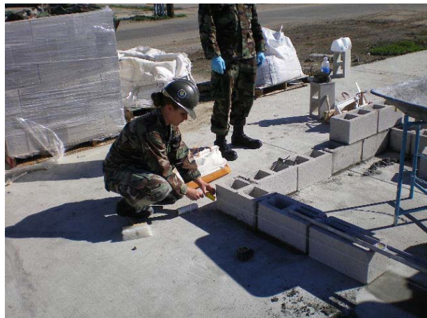
Figure 8-20 – Checking for alignment.
