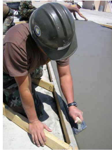
Figure 6-73 – Edger in use.
