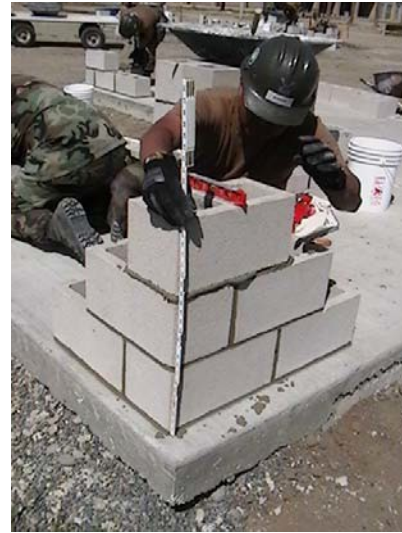
Figure 8-23 – Using a folding rule to check course height.
