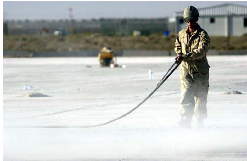
Figure 6-78 – Sprinkling concrete with water.
