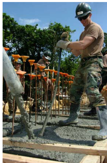
Figure 6-63 – Using a vibrator to consolidate concrete.
