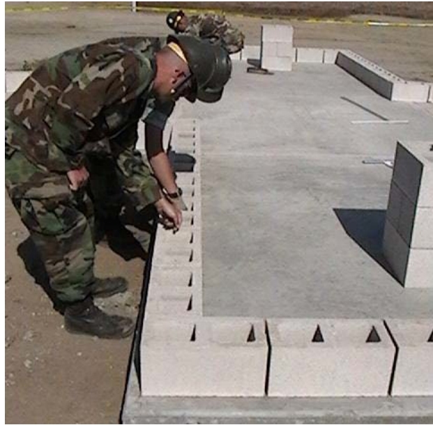
Figure 8-13 – Placing blocks without mortar (chasing the bond).
