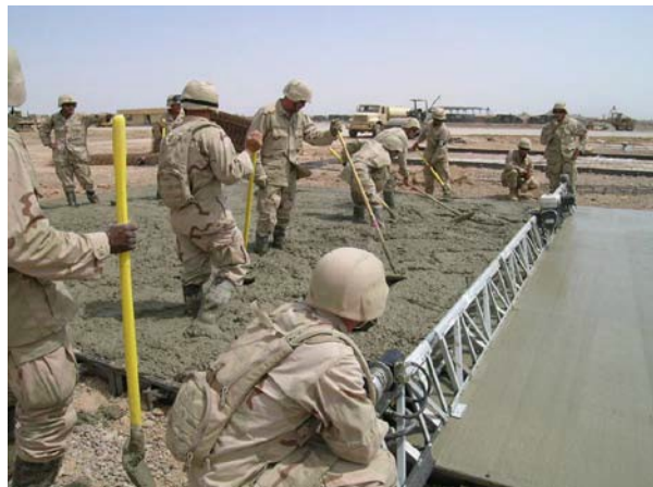
Figure 6-66 – Mechanical screed.
