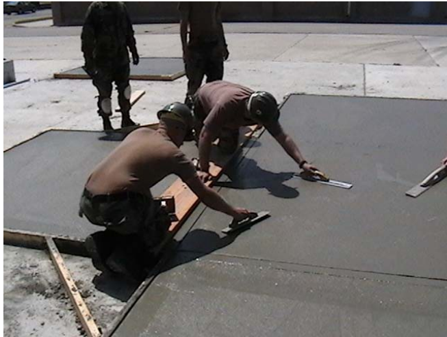
Figure 6-70 – Hand float in use.
