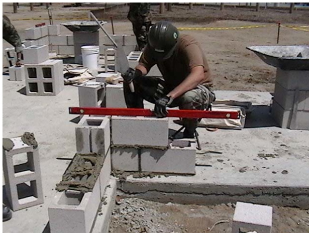
Figure 8-21 – Checking for level.
