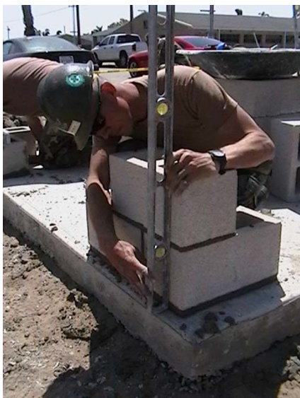
Figure 8-18 - Plumbing block for a wall.
