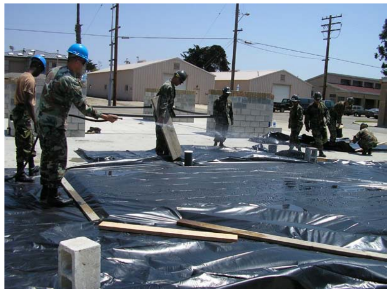
Figure 6-79 – Curing concrete with plastic.
