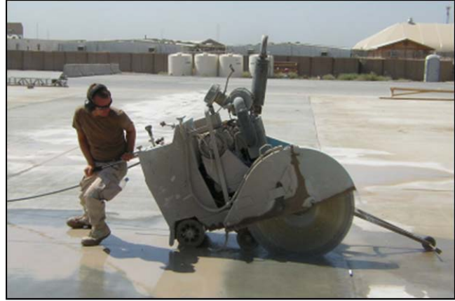
Figure 6-61 – Concrete saw.
