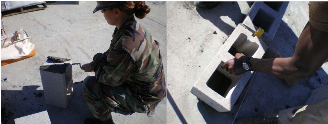
Figure 8-16 – Laying first course of blocks for a wall.
