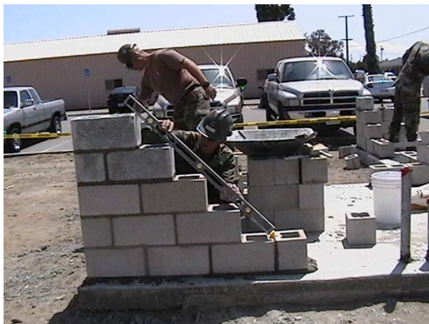
Figure 8-24 – Checking horizontal block spacing.
