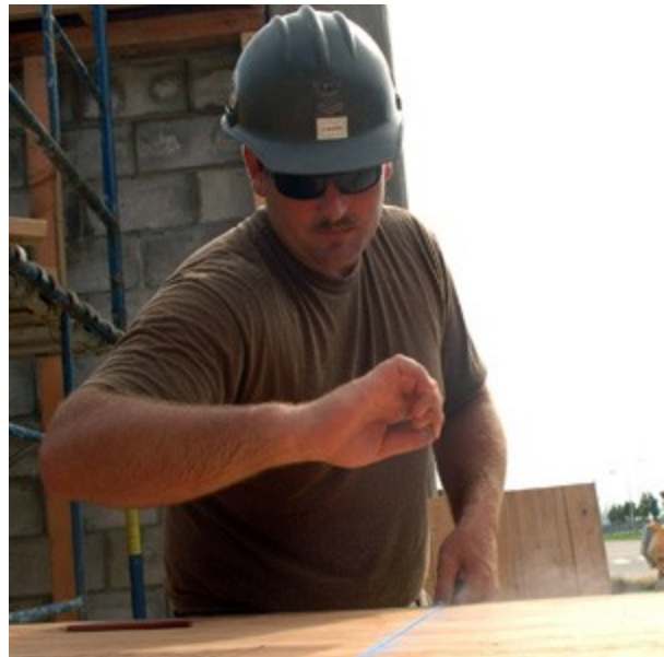
Figure 2-16 Proper use of a chalk line.
